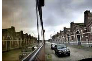
The architectural firm hopes to revive the old warehouses with, among other things, a large indoor market.
