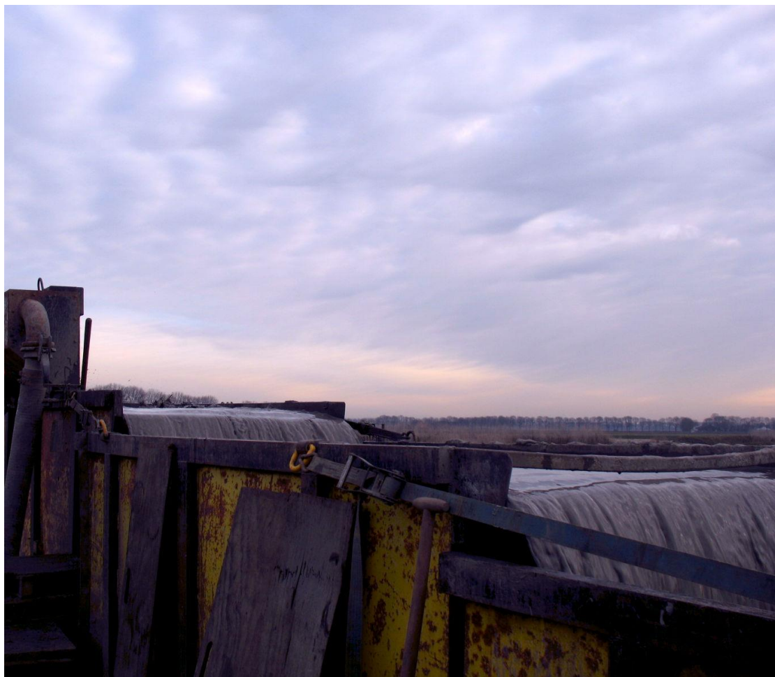
Fig. 2: Water removal during drilling
