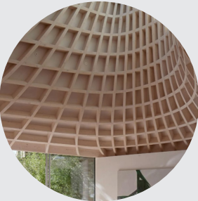
Locally Sourced Wood Ribs
