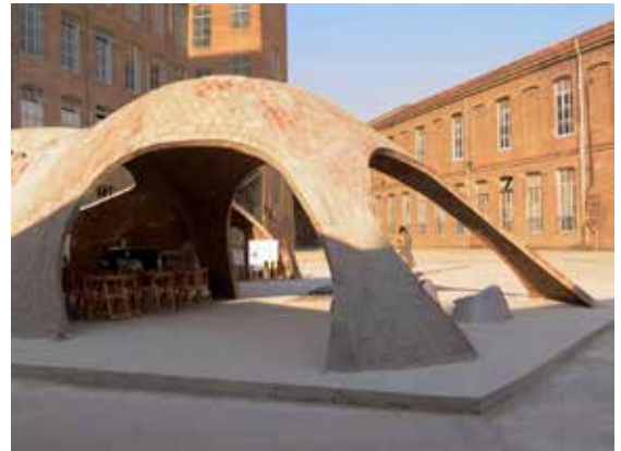
Image 17 & 18. Bricktopia pavilion designed with Rhinovault (Block13, 2014)
