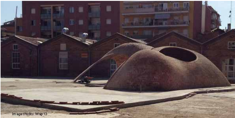
Image 17 & 18. Bricktopia pavilion designed with Rhinovault (Block13, 2014)
