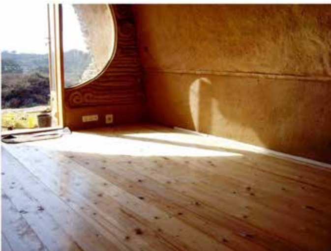
Image 19 & 20. Tamera eco-village in Portugal, built with rammed earth (Open Source Ecology, 2014)
