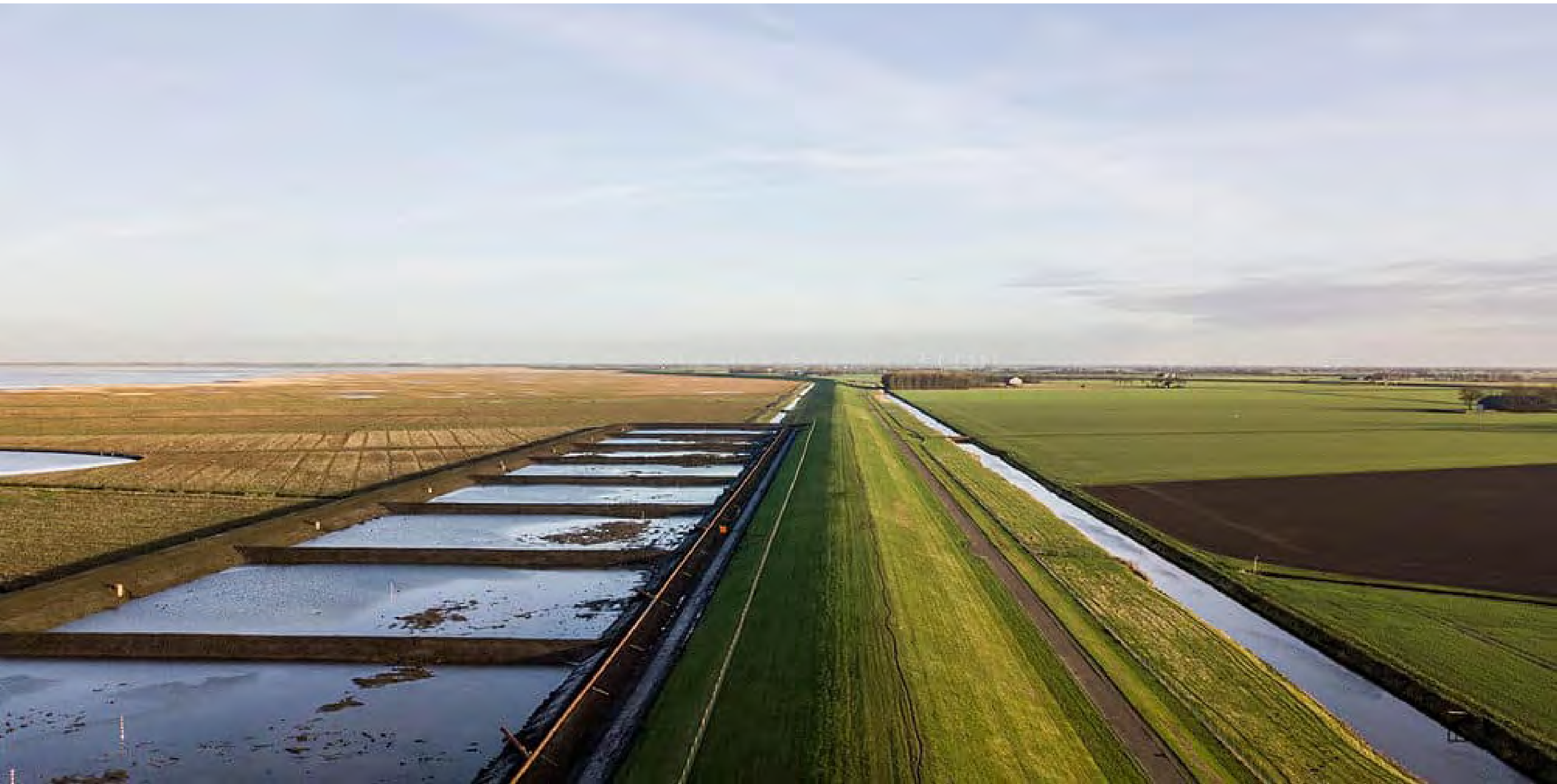
Brede Groene Dijk : A dike made of salty dredging sludge Photo: Elcke Vels, 2022
