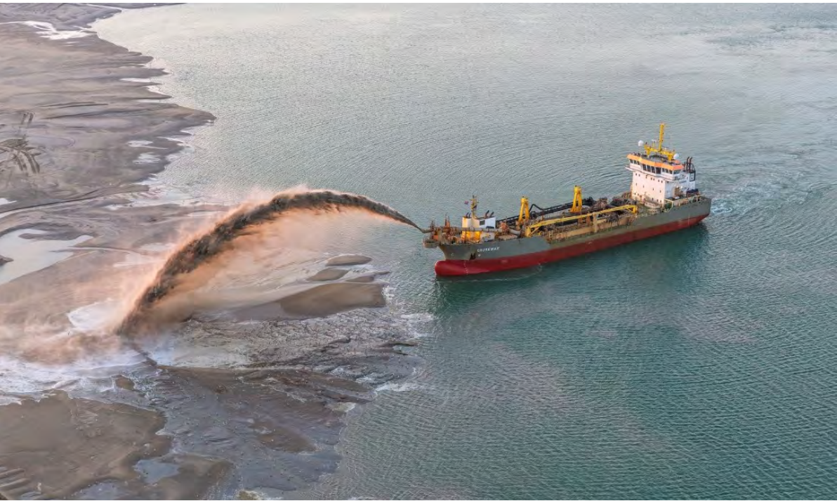
Replenishments, dredging and pumping sand onto beaches. Photo: Zlatan Hrvacevic, 2022.
