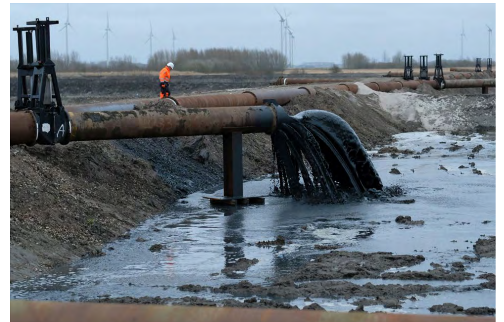
Raising sludge by pipeline in plots with ring dyke. Image of clay mill. Source: Christiaan van Velzen, 2018
