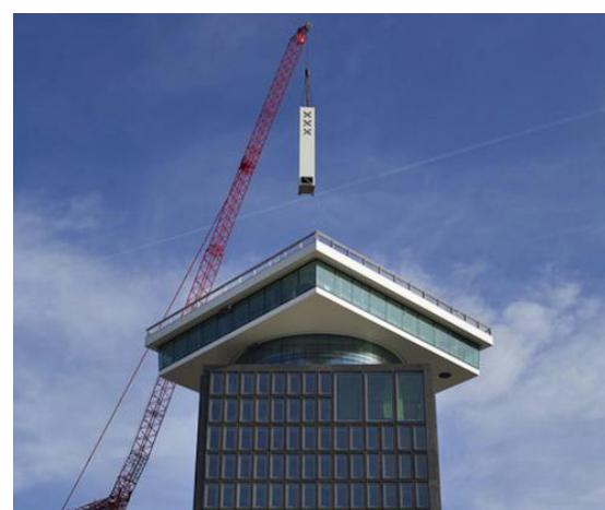
A'Dam tower. Crown installation<sup>5</sup>
