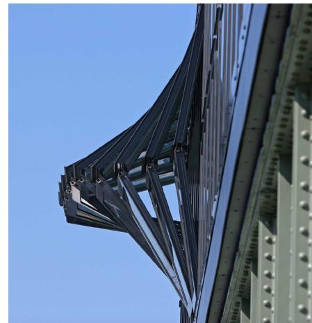
organized a design competition in 2005 and the entry by de Architekten Cie. was chosen from the 14 submissions. OPEN café-restaurant is a pure, transparent, glass volume that fits precisely onto the existing bridge. It is composed of a floor, a roof and a glazed façade that is formed entirely of pivotal windows, all of which can be opened.
