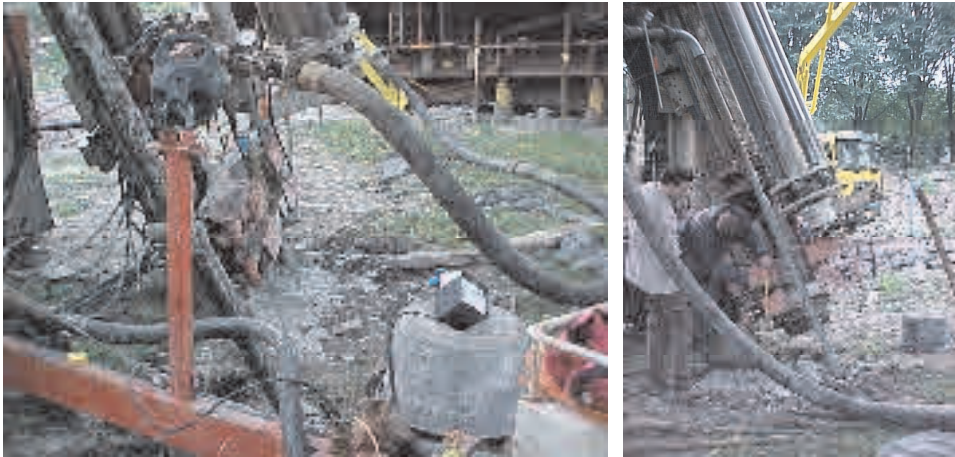
Figure 6.20 Cement Bentonite Sleeve Grout Backflow at Surface Level
