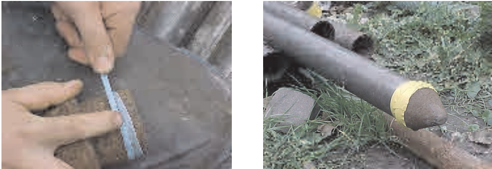
Figure 6.17 Attachment of a Removable Plug at the Bottom End of the Tube
