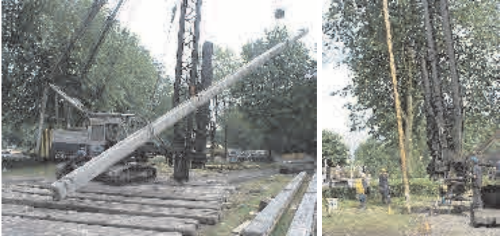
A. Figure 1 Driving of Concrete ( left ) and Wooden ( right ) Piles
