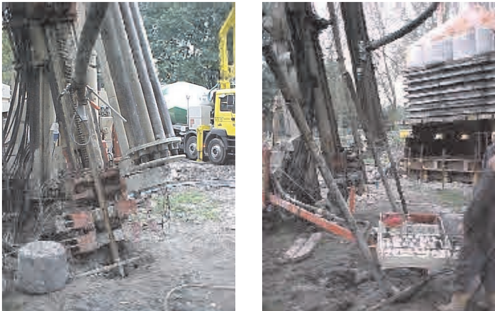
Figure 6.18 Installation of the Tubes
