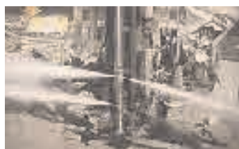
Figure 5.1 Jet Grouting: High Pressure Cutting with Water (Shown at Surface Level)
