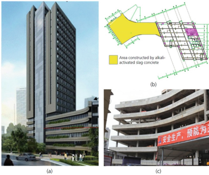
Fig. 14 Alkali-activated slag demonstration project: a building; b construction section; c side view of the structure made with alkali-activated slag concrete [17]. Foto archive of Prof. Caijun Shi
