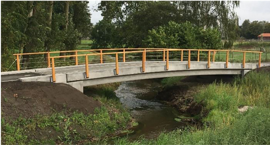
Fig. 11 Bicycle bridge in The Netherlands. Foto archive of Martin Verweij
