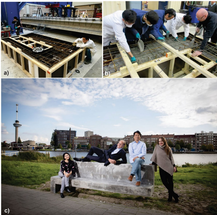
Fig. 3 a Preparation of the pre-casting model, b pouring the alkali activated concrete and c the final concrete bench [4]. Photo archive of TU Delft
