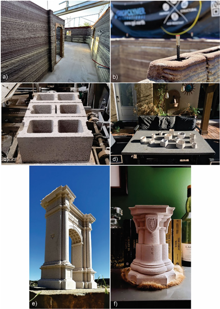
Fig. 21 a and b first 3D printed house out of geopolymers constructed in Amargosa Valley, Nevada in the spring of 2023 by Geopolymer International in collaboration with StrongPrint3D and Renca, c GeoBlock (MK-based) used for walls, as well as arches and domes, d GeoCement (MK-based) used for a variety of casting and spraying purposes including structural concrete, ornamental items, and repairs or fireproof coating [35]
