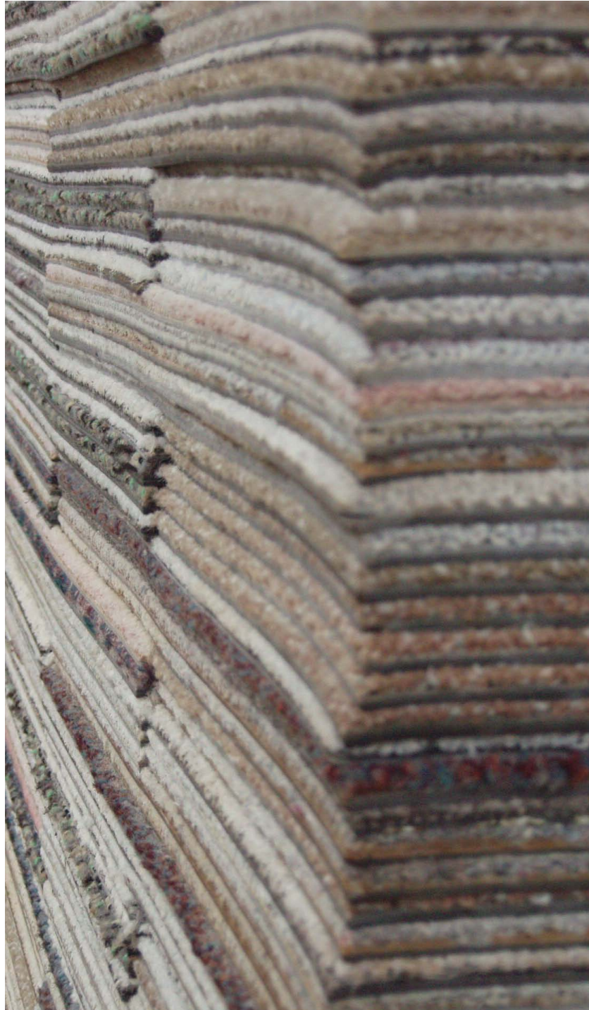
Tiles stacked as walls, held in compression by wooden ring
