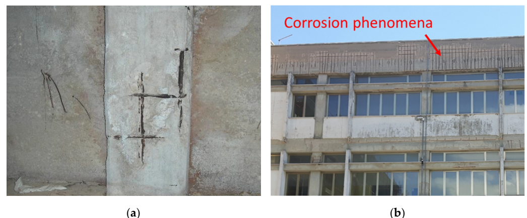
Figure 6. Example of corrosion phenomena to a column in the basement (a) and façade structural members (b) observed during in situ surveys (from UEFA/ELENA research project [23]).
