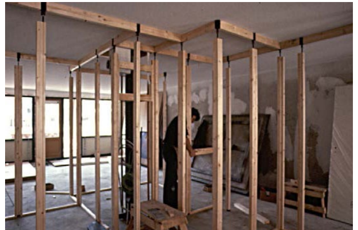
Fig. 3.6: During installation of the infill package. Showing the fixed position of staircase and central shaft, along with the structure of the adjustable partition walls. From: Lunetten 4D , by Frans van der Werf, 2017.
