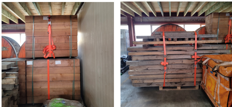
Figure 5.4: Dunnage Piles observed at yard
