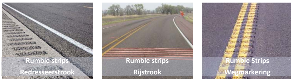
Figuur 13 Rumble strips (Bronnen van links naar rechts: Moloco, U.S. Department of Transportation, Just Drive PA)
