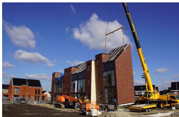
Figure 9 Placement of a Startblock unit (Startblock, n.d.-a).
