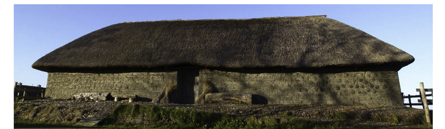
Fig. 2.8. Top : A recently repaired turf wall made of clamped blocks at Tyrfinnsstaðir. Bottom : Experimental reconstruction of an early-medieval turf house on a turf platform in Firdgum. Photo © D. Postma.
