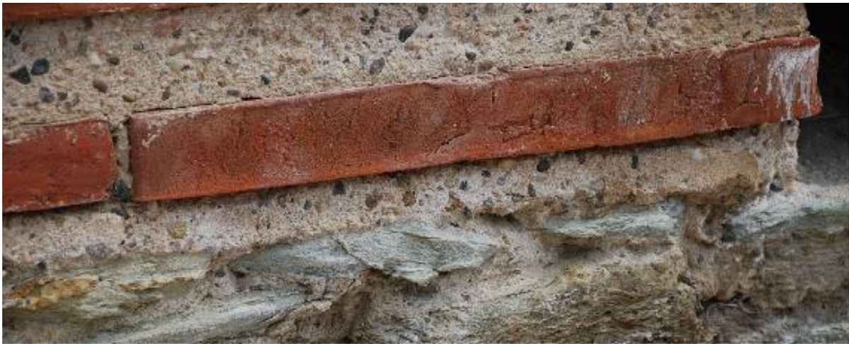
Fig. 30 Repair mortar in a mix structural system of Galerius Palace in Thessaloniki, Greece
