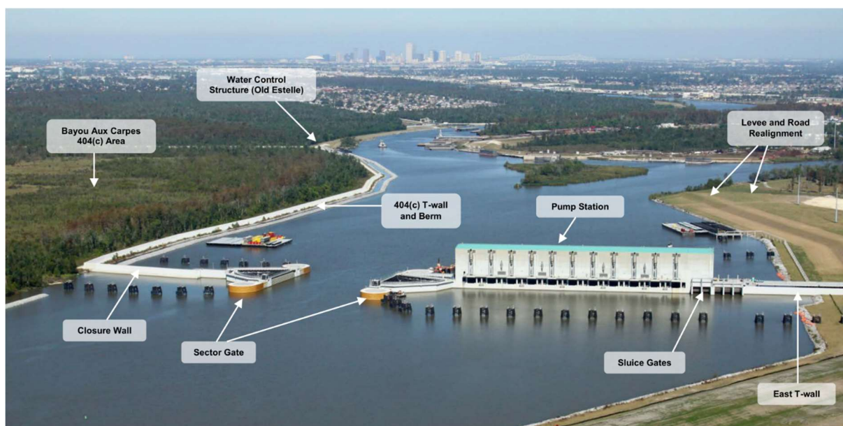
Figure ii.2 Overview of the West Closure Complex project. From U.S. Army Corps of Engineers (2013, p. 2).
