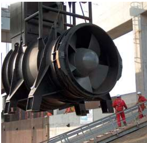
Figure ii.4 (left) Front view of one of the newer axial-flow pumps of IJmuiden (NGS, n.d.).
