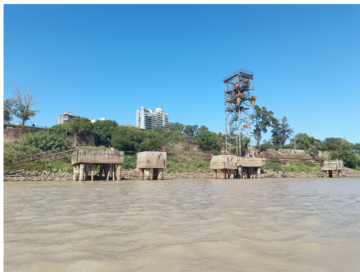
Figure 5.9: Structure in front of Parque de Las Colectividades
