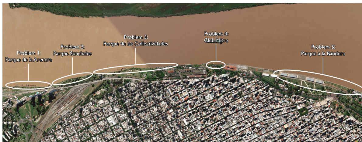
Figure 3.2: Overview of the embankment problems
