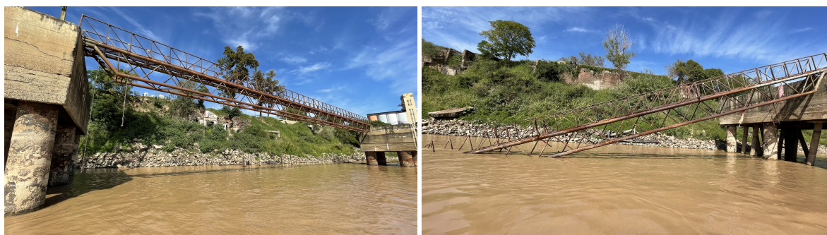
Figure 5.14: Bridges between the dolphins
