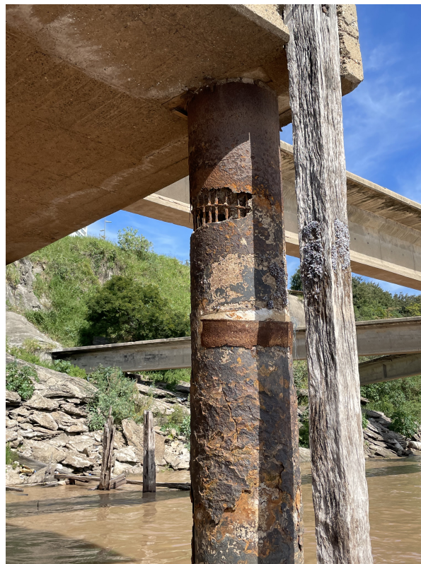
Figure 5.7: Close-up supporting pile
