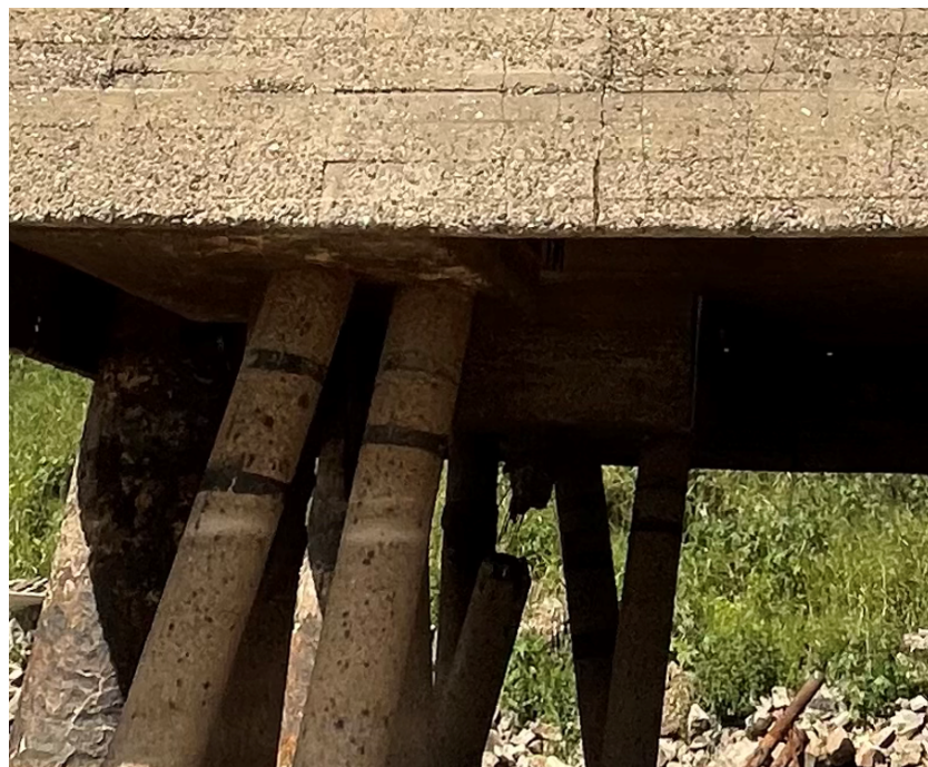
Figure 5.13: Foundation grain tower
