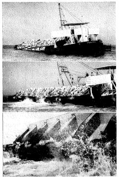
New methods and new materials had to be proved for the execution of the Delta Plan. This floating mechanical way of plunging masses of stones proved to be a success.
