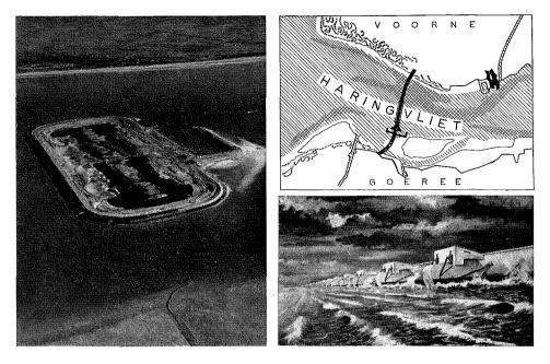
Closing off the Haringvliet estuary. Left the gigantic pit for the seventeen discharging sluices under construction. Right on top the situation, below the planned complex of sluices.
