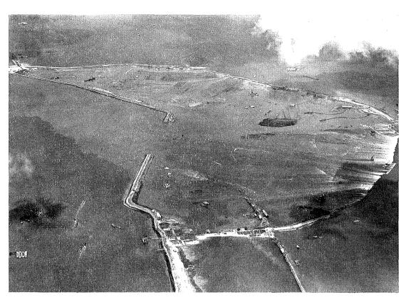
The breach of the dike at Schelphoek, Schouwen (seen at the left) was closed by means of a ringdike, 2.65 miles long, 235 concrete boxes,  $36 \times 23 \times 23$  ft. and 1 Mulberry pontoon of 7000 tons were used plus 2,200,200 sq.ft. of willow mattresses.
