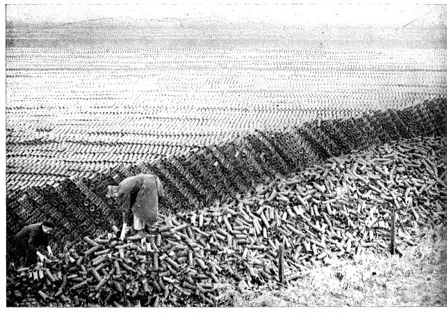
DRAINAGE TUBES FOR THE ZUIDERZEE RECLAMATION The heap shown here represents only a very small fraction of the drainage tubes needed. (*Photo A.N.P.*)
