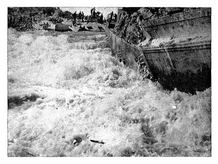
Enclosure of one of the gaps of Walcheren by means of scuttled ships. The fierce currents have broken the ship and find their way underneath it.
