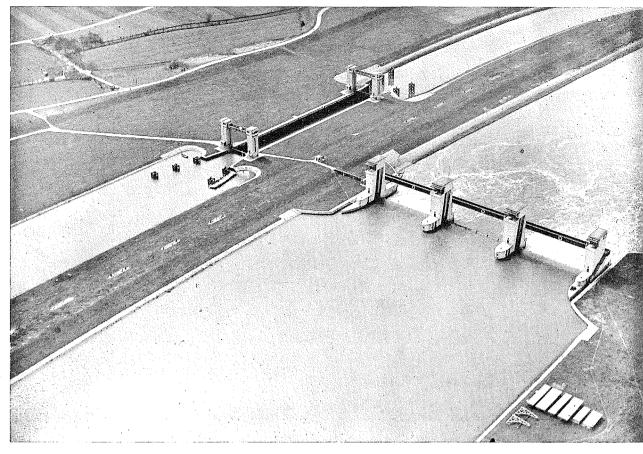
Weir and lock in the canalized Maas. The lock is for 2000-ton ships.
