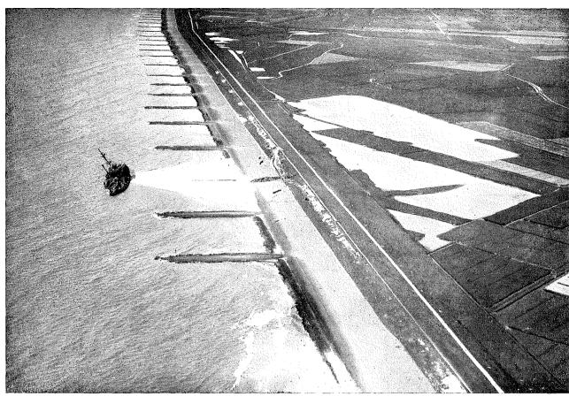
COASTAL DEFENCE BY MEANS OF STONE GROYNES AND A STRONG DIKE A ship has stranded. Behind the dike a lake was formed by removing the substance needed for the dike. (Photo K.L.M.)
