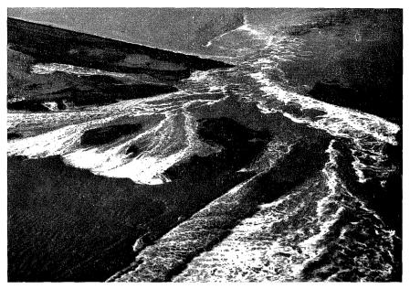
Ebb-current through a breach in a dike, February 1953. Tidal gullies cause small waterfalls, which erode backwards. Those gullies thus lengthen, widen and deepen daily, the sand in the soil is being swept either into the sea or is deposited on the inundated lands. The storm of 1953 created 76 of such stream-carrying breaches.
