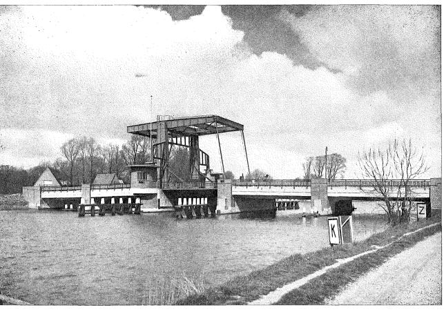
Typical Dutch movable bridge across a canal, allowing quick passage of ships.
