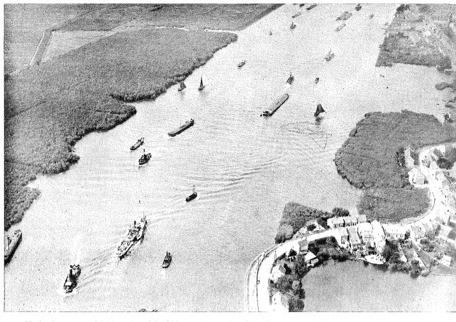
Navigation on one of the branches of the Rhine near Rotterdam. The dike with the road upon it serves as a foundation of houses as well. In the foreground a repaired ancient breach. (Photo K.L.M.)
