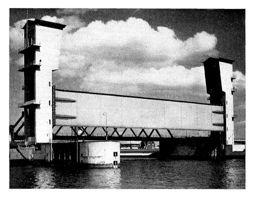
The latch on Holland's front door. This movable storm flood defence in the Hollandse IJssel was Delta work number one. In the above picture it is seen from the sea side; below the gate in closed position.
