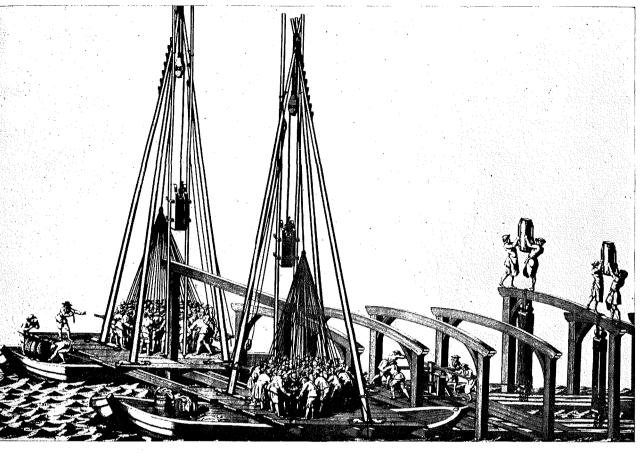
BUILDING IN MORASS AND WATER by means of wooden piles, (Picture from about 1700).
