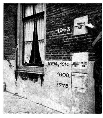
Flood-stones, indicating the levels to which floods rose, in buildings standing at the shores of tidal inlets, give us an idea of how these buildings settle. Dikes settle more because heavier.
