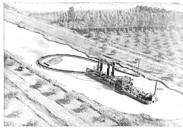
SUCTION DREDGE making a canal. The dredgings are pumped through a floating tube to the dump. (Photo K.L.M.)
