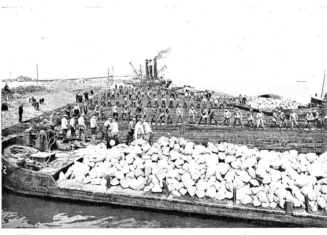
Willow mattresses being sunk with stones to prevent scouring of the new dike. In the background a floating pumping station, which pumps sand to make the dike. (Photo Maaskant)
