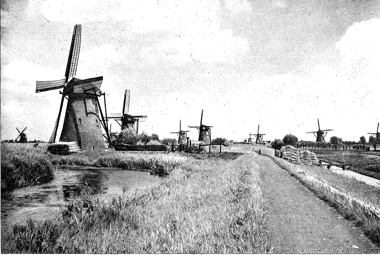
At Kinderdijk, near Rotterdam, windmills, pumping the surplus water out of the country, are still abundant. Streamlining and ball bearings are the modern means to make them more efficient. (Photo J.G. van Agtmaal)
