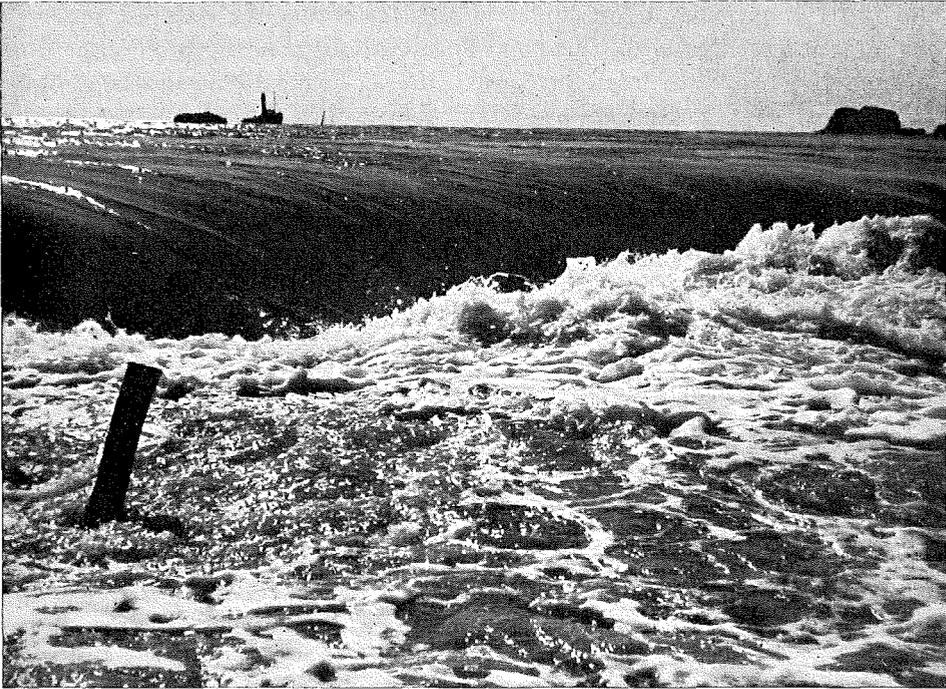
Strong tides in the breaches of Walcheren, causing waterfalls of more than 4 feet. The soil consists of loose sand, upon which willow mattresses have been laid. *(Photo Henning)*
