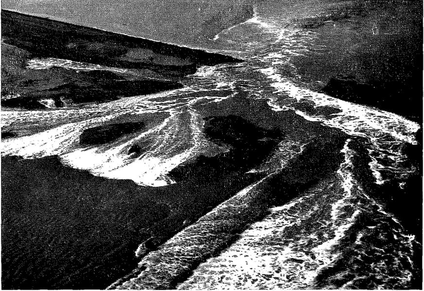
Ebb-current through a breach in a dike, February 1953. Tidal gullies cause small waterfalls, which erode backwards. Those gullies thus lengthen, widen and deepen daily, the sand in the soil is being swept either into the sea or is deposited on the inundated lands. The storm of 1953 created 76 of such stream-carrying breaches.
