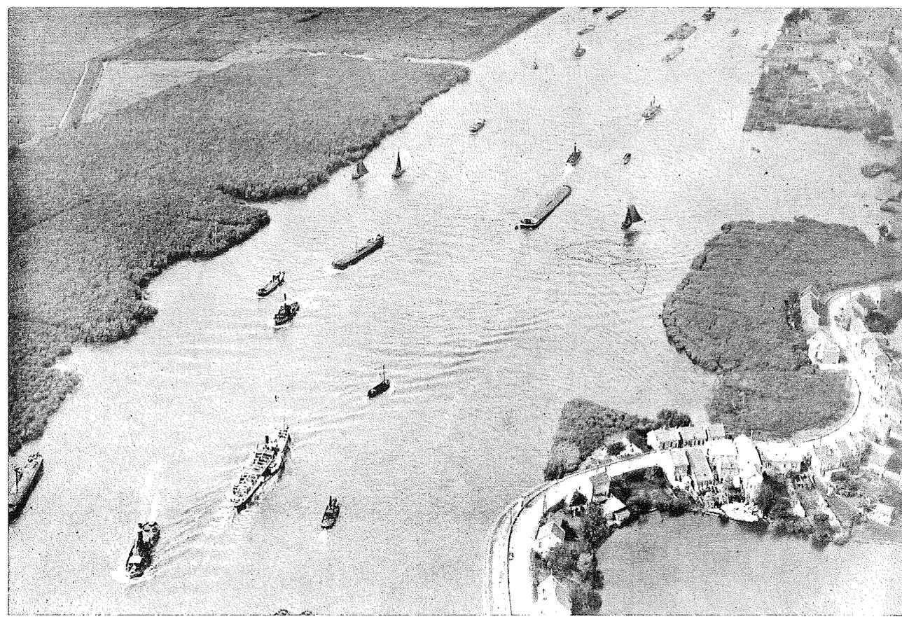
Navigation on one of the branches of the Rhine near Rotterdam. The dike with the road upon it serves as a foundation of houses as well. In the foreground a repaired ancient breach. *(Photo K.L.M.)*
