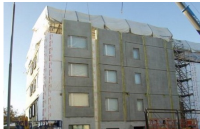
Figure 50. Attaching prefab. panels Source: http://www.ttu.ee/
