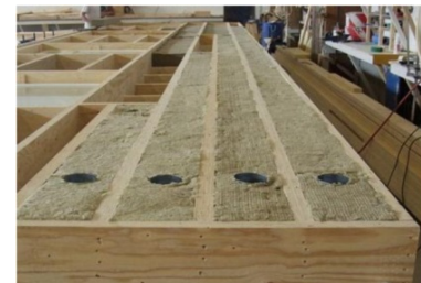
Figure 51. Wooden frame filled with rock wool and ventilation shafts Source: http://www.ttu.ee/
