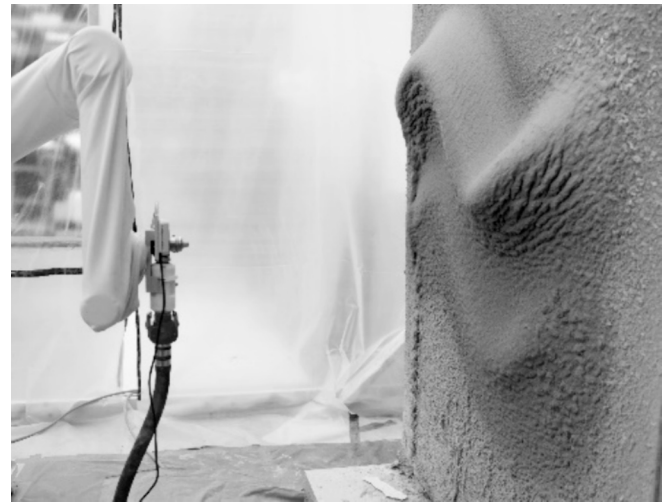
Fig. 6. Robotic Plaster Spraying (RPS) introduces a gravity-resisting, vertical thin-layer spray-based printing technique (ETH Zurich, 2021) [30].
