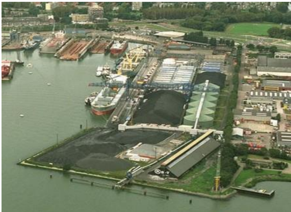
Figure 3.15: Rotterdam Bulk Terminal aerial view (Image courtesy of RBT B.V.)
