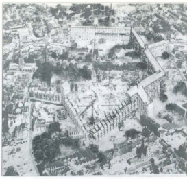
Golden Lane Housing Prototype van Alison en Peter Smithson gemonteerd in de gebombardeerde Coventry \ Alison en Peter Smithson's Golden Lane Prototype superimposed on bombed-out Coventry (uitfrom: Kenneth Frampton, 'The Generic Street as Continuous Built Form', in: Stanford Anderson (ed.), On Streets , 1978)
