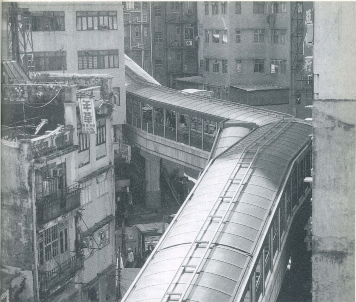
Voetgangersbrug in Hong Kong \ Pedestrian bridge in Hong Kong (fotofoto: Mapoffice)
