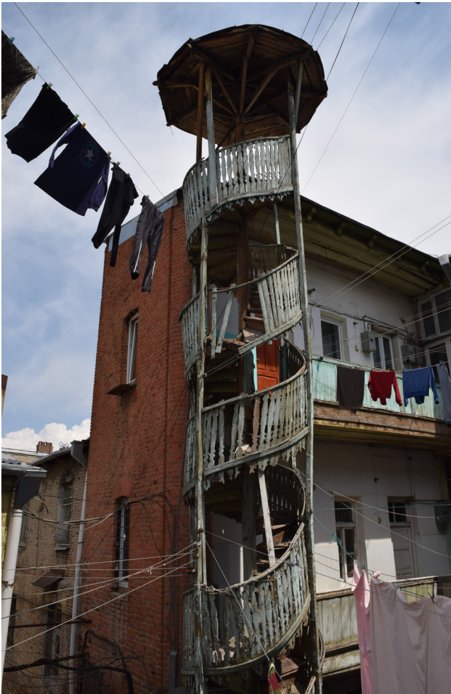
Fig. 18 Tbilisi. The Staircase before the conservation project. The residents were using it on a daily basis even though near collapse.
