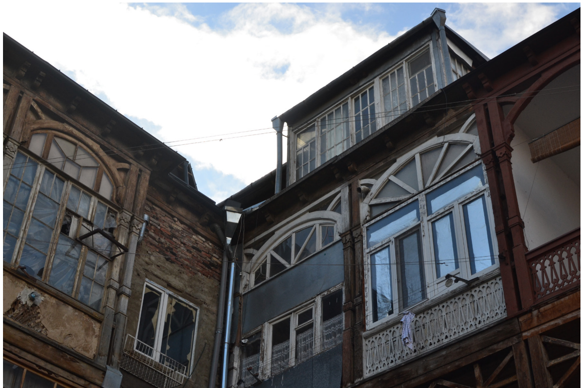
Fig. 9 Tbilisi. Some fractions of the loggias have been closed to enlarge the space of the house in a typical courtyard house.
