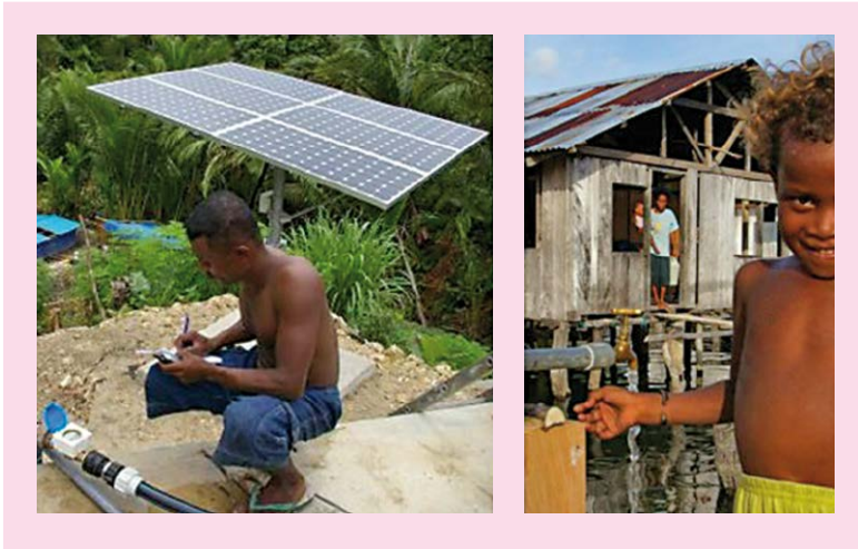
Figure 1.3 A solar pump provides clean water to a village (PicoSol, 2014)
