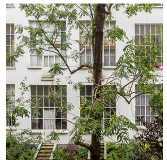
The atelier facade
