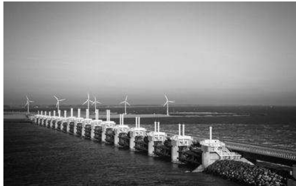
Figure 1.2: The Eastern Scheldt storm surge barrier, or Oosterschelde. (photo by Rob Broek/iStockPhoto.com)
