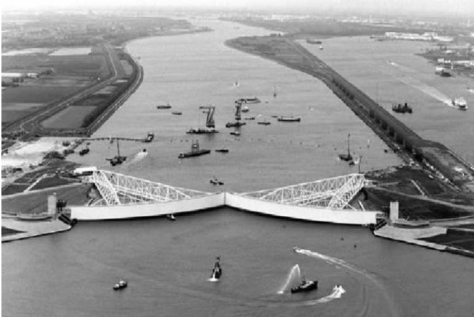
Figure 1.3: Storm surge barrier at the New Waterway. (photo taken from Microsoft Encarta Online Encyclopaedia 2008)
