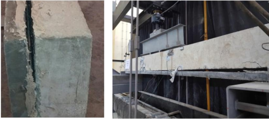
Figure 2.19 Debonding at the interface [23,96].
