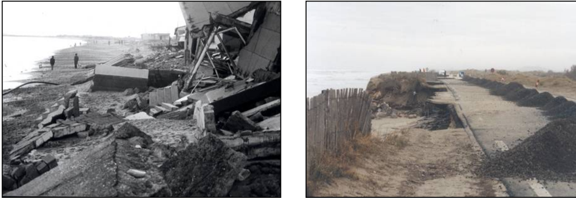
Figure 46. Destruction caused by the 1982 storm.
