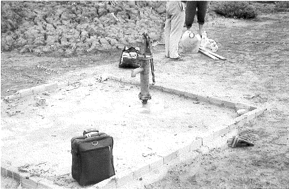
Picture 5: Steel pump with the concrete foundation. The white spot made on the on the pump was chosen to be the zero-level for the leveling, the reference level.
