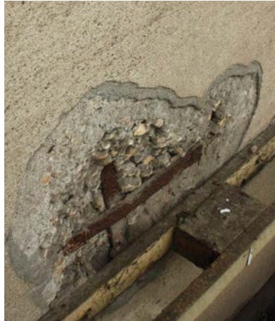
2 Corrosion of the reinforcement
