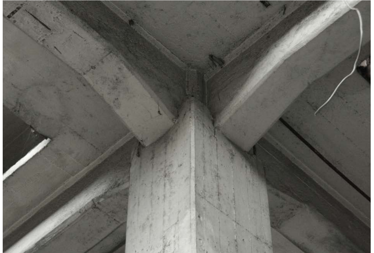
Beam column connection
