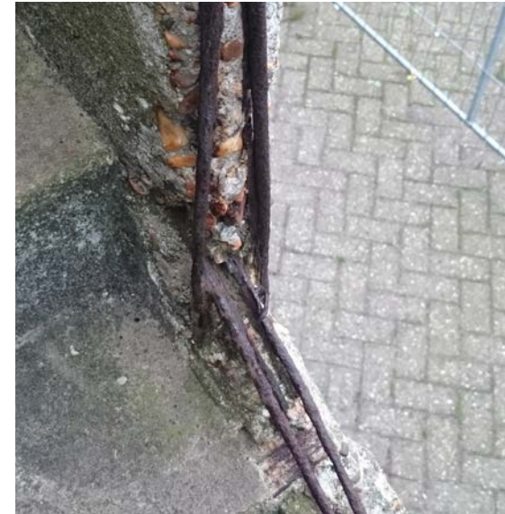
Image 3 - Reinforcement of exterior stair.
