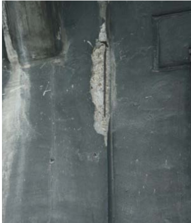
1 Spalling of concrete
