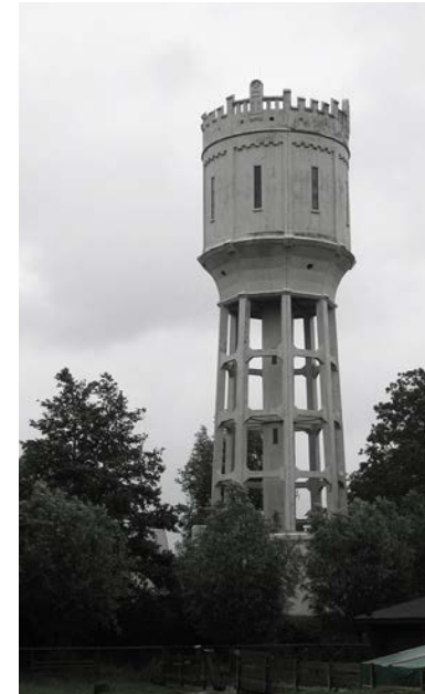
2. Early example of a reinforced concrete watertower
