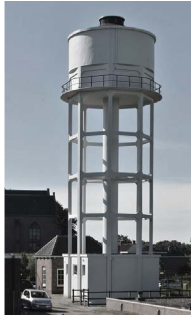
1. First open structure water tower
