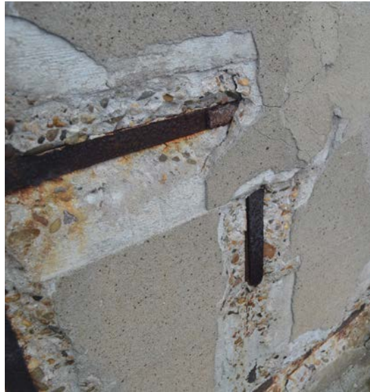
Image 2 - Wall reinforcement.
