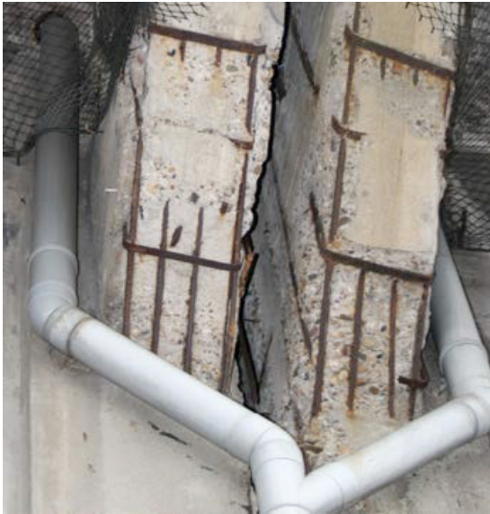
Image 1 - Typical reinforcement of the Hennebique system with horizontal strips.
