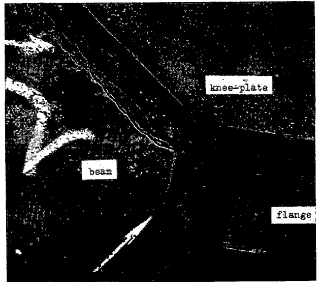
Fig. 50. Crack in beam at point B of no. 42 (dynamic tension)
