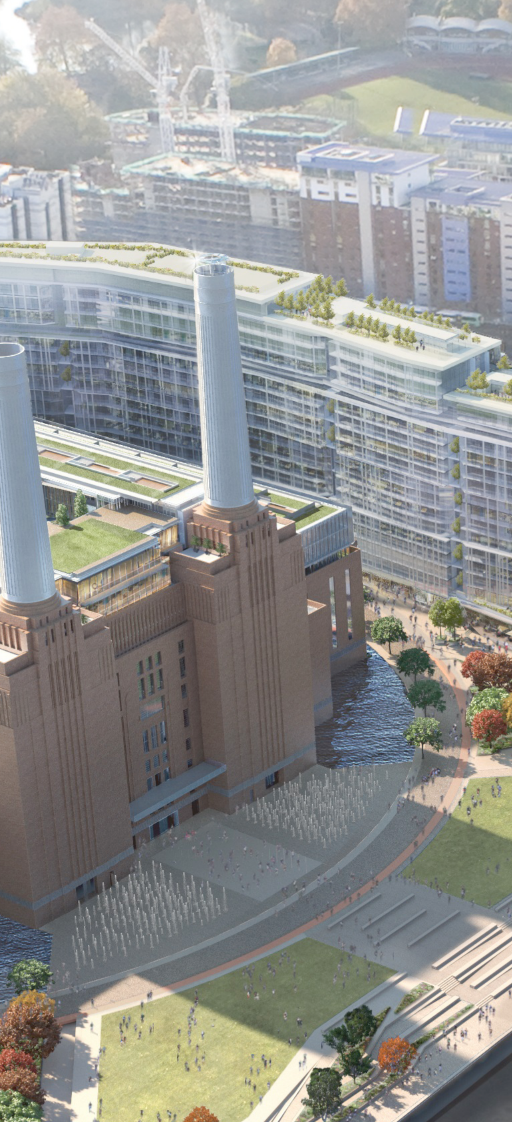
Battersea area reconstruction project. Source: https://metrouk2.files.wordpress.com/2014/10/battersea-thames-pic.jpg
