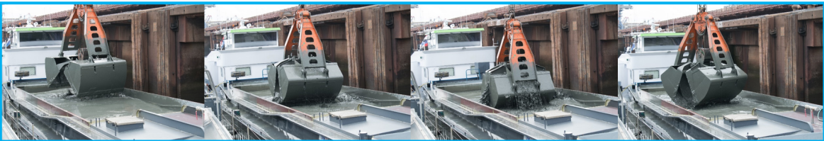
Figure 3.13: Mixing the mud with backhoe to make it homogeneous.
