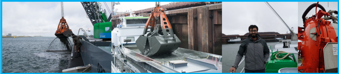
Figure 3.11: The fluid mud dredged at Calandkanaal (Port of Rotterdam) and transported it by truck to the flume at Deltares.
