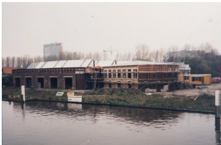
Figure 25 De Beuk under construction, November 1996. Source: (ProteusEretes, n.d.)
