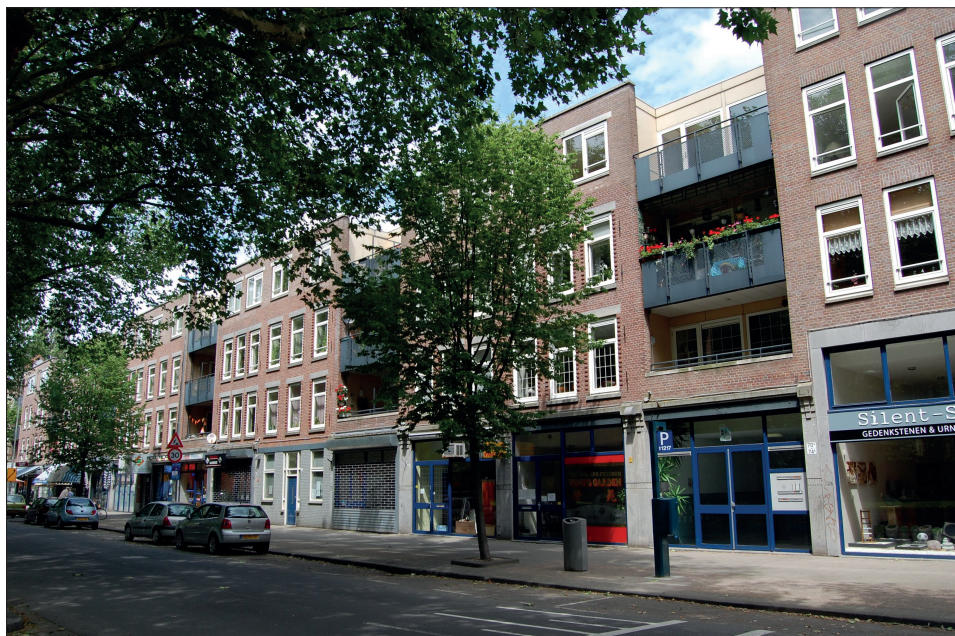
Fig. 5. Saved from demolition
