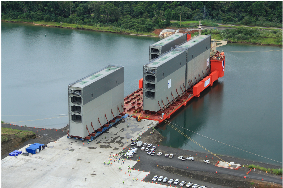
Figure 3.1: Sea lock gates for the new Panama canal [23].
