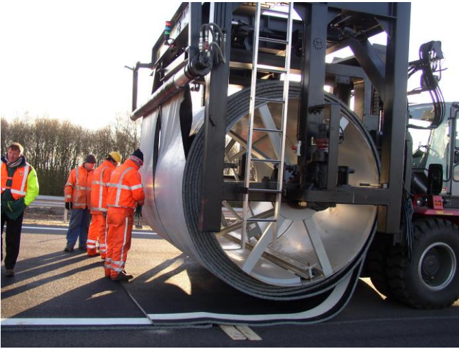
Fig. 4: Rolled up asphalt concrete
