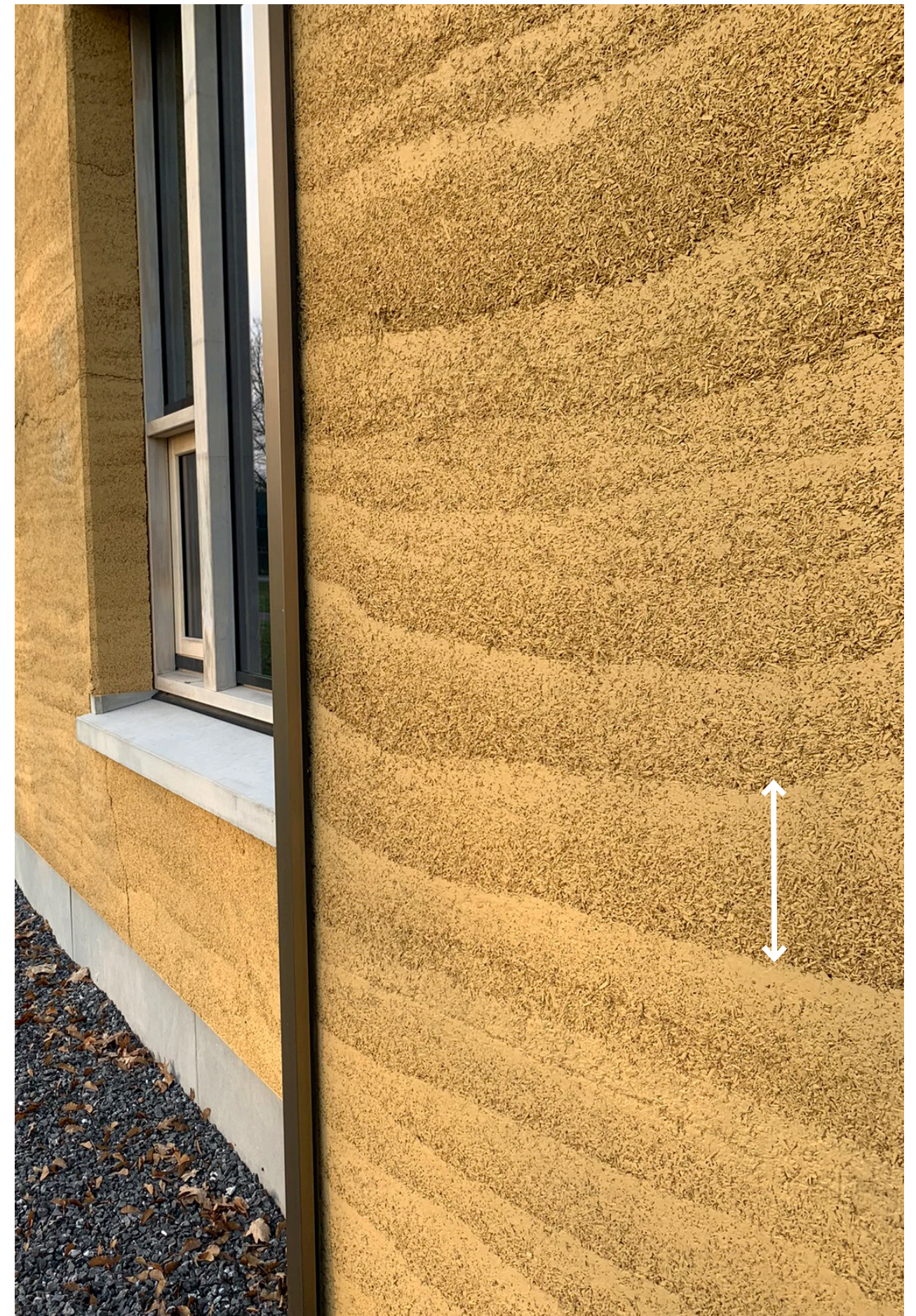
Fig 4.9 Uncontrolled layer height and clear density gradient
