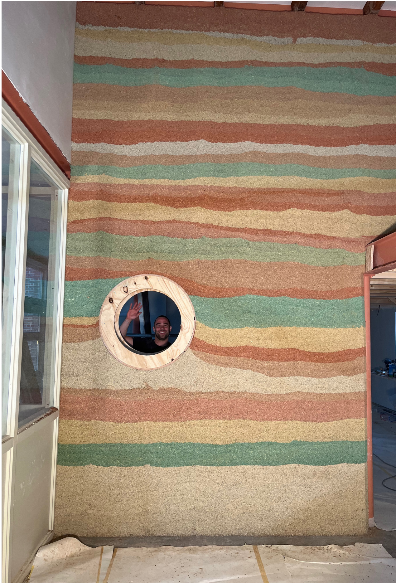
Fig 4.16 Cast-in situ hempcrete wall. Project by HOP Architects and YOMABOUW
