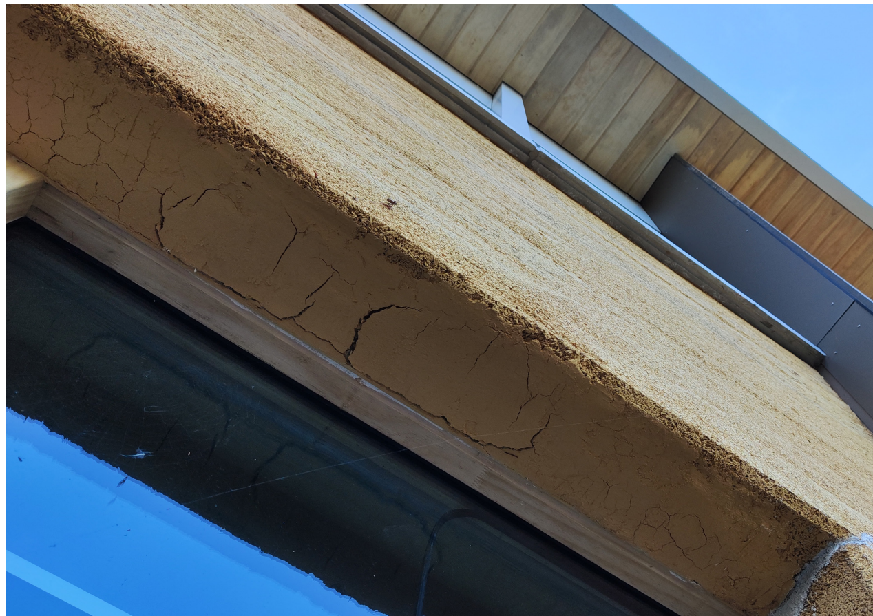
Fig 4.8 Cracks at window frame
