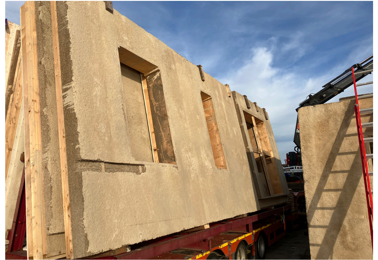
Fig 4.14 Prefab hempcrete system, shipped to site on a trailer
