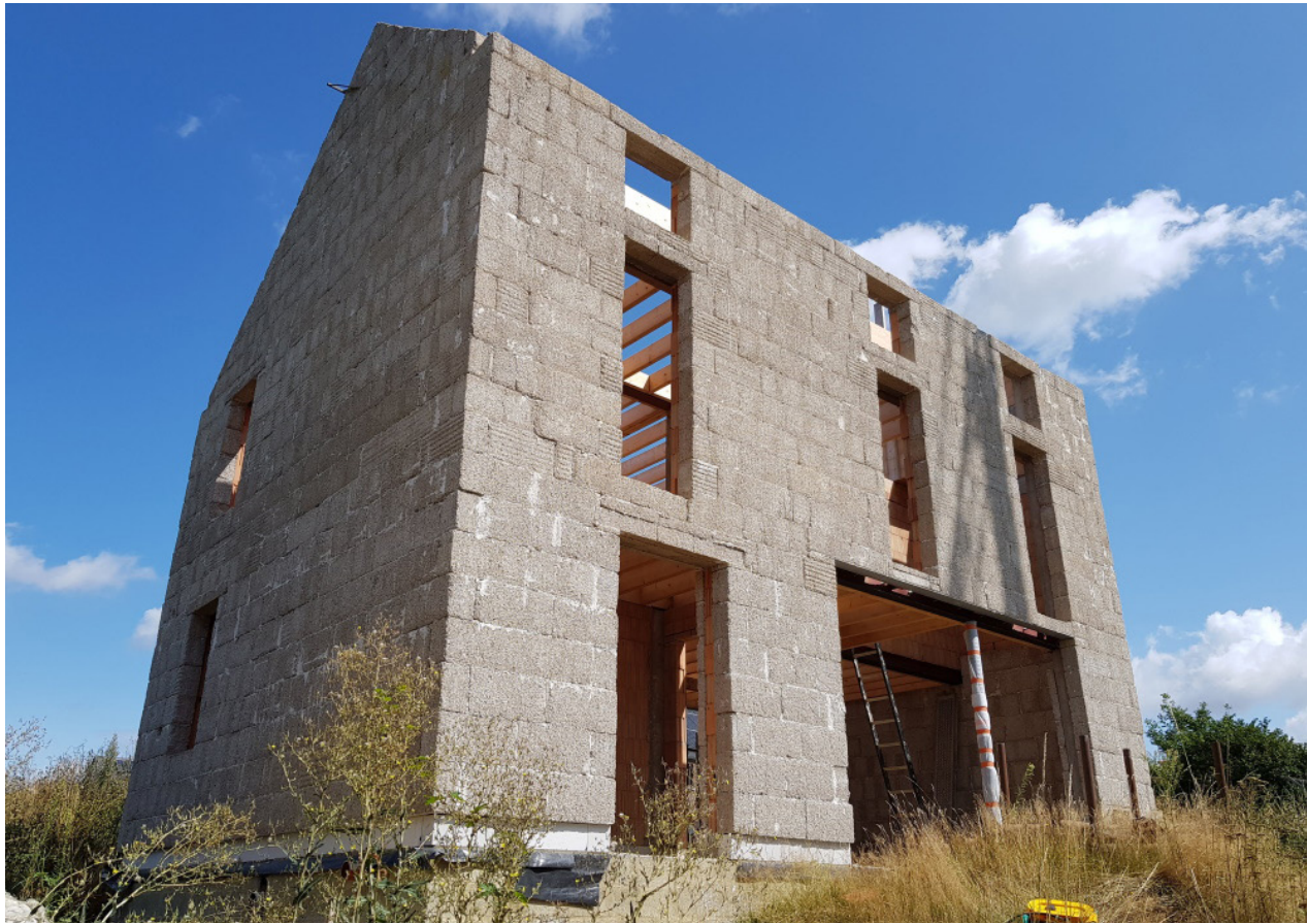
Fig 4.12 Stacked IsoHemp block wall, non load bearing
