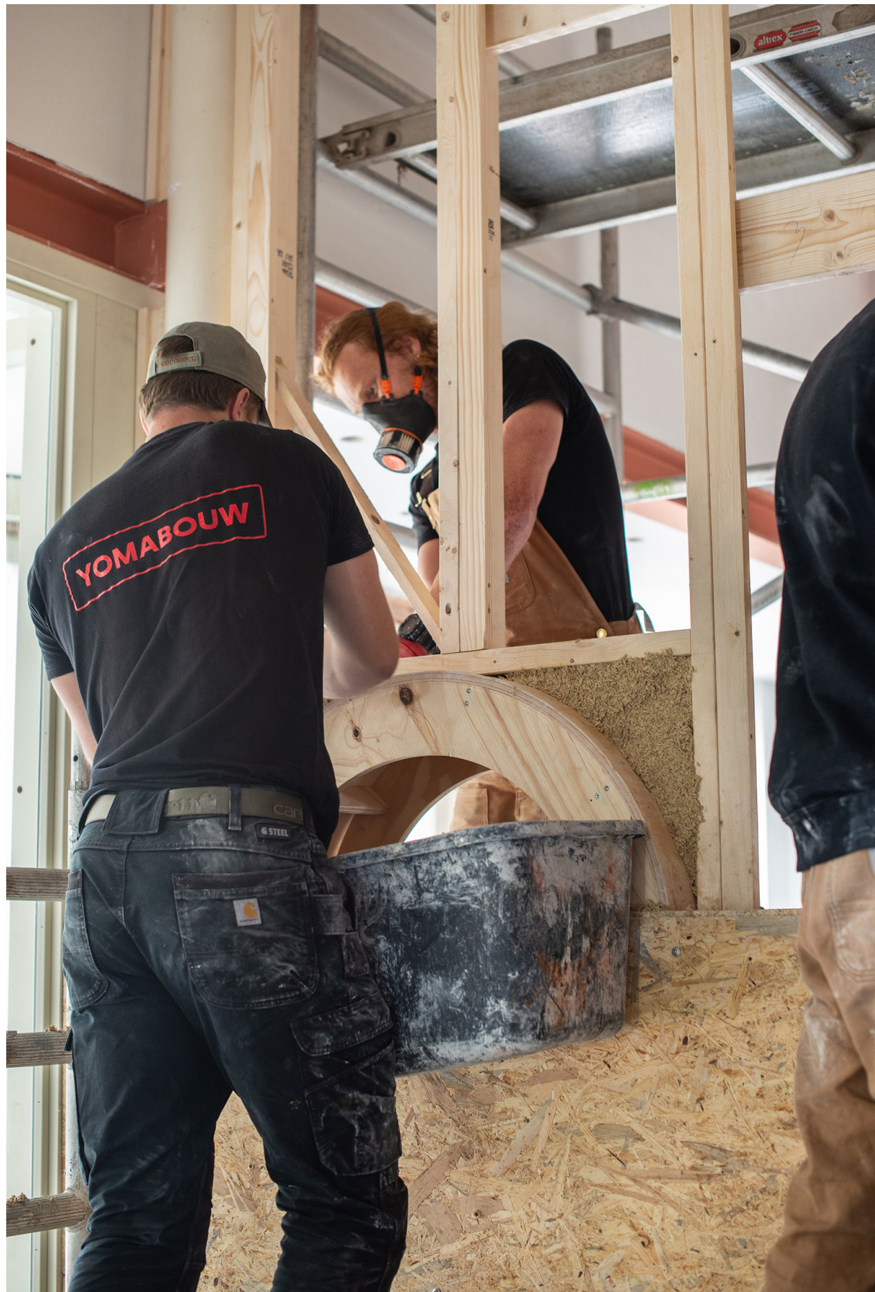
Fig 4.6 Manually placing the hempcrete in the formwork
