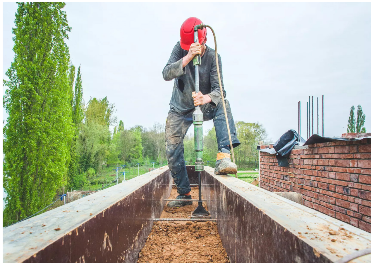
Fig 4.17 Worker using a pneumatic rammer to construct a rammed earth wall
