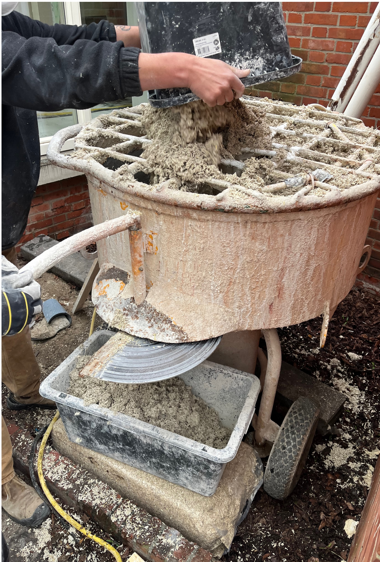
Fig 4.4 Mixing and filling the tubs
