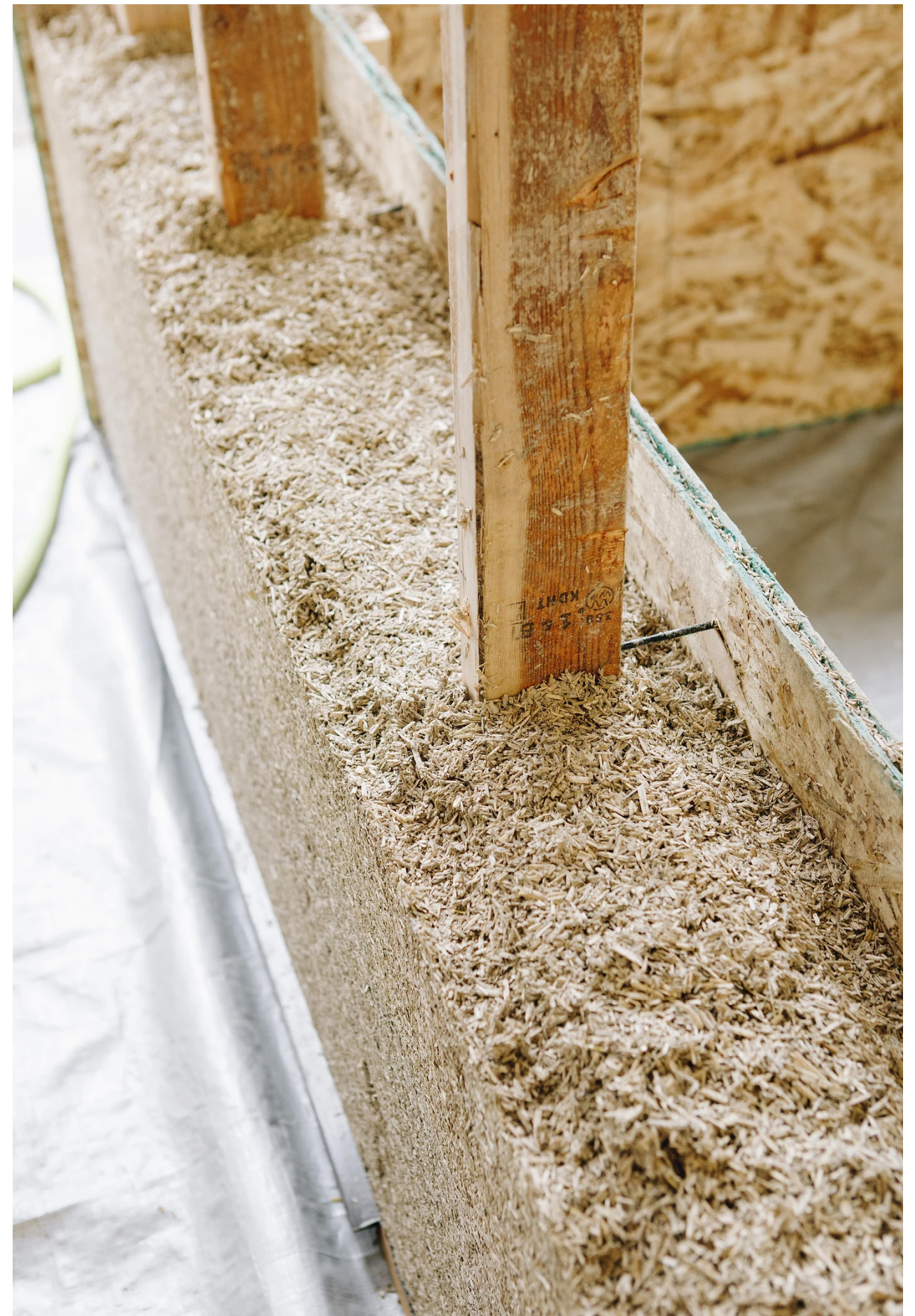
Fig 2.15 Exposed hempcrete facade. Formwork is removed, studs account for load
