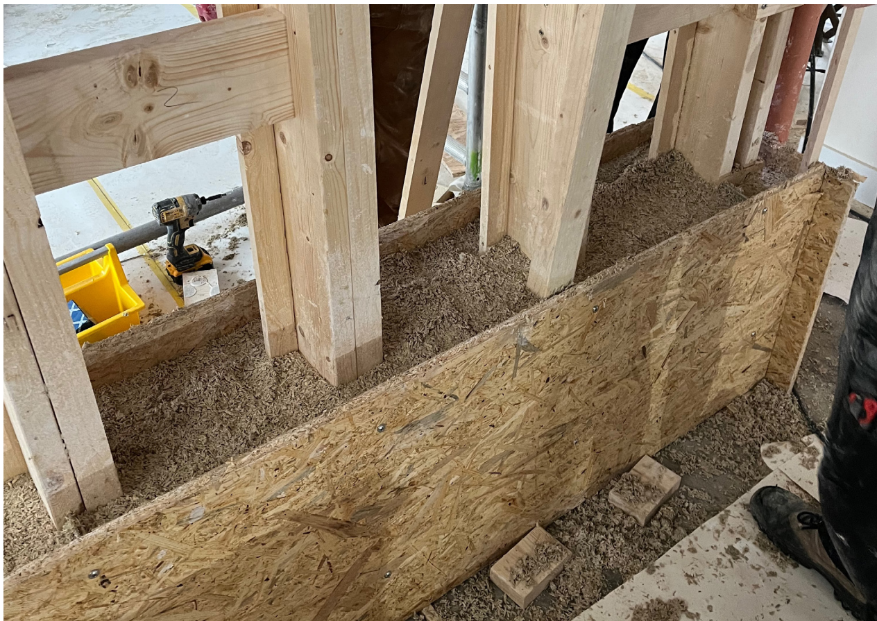
Fig 2.14 Building of a Hempcrete wall: Cast-in-situ around a wooden stud frame using a formwork
