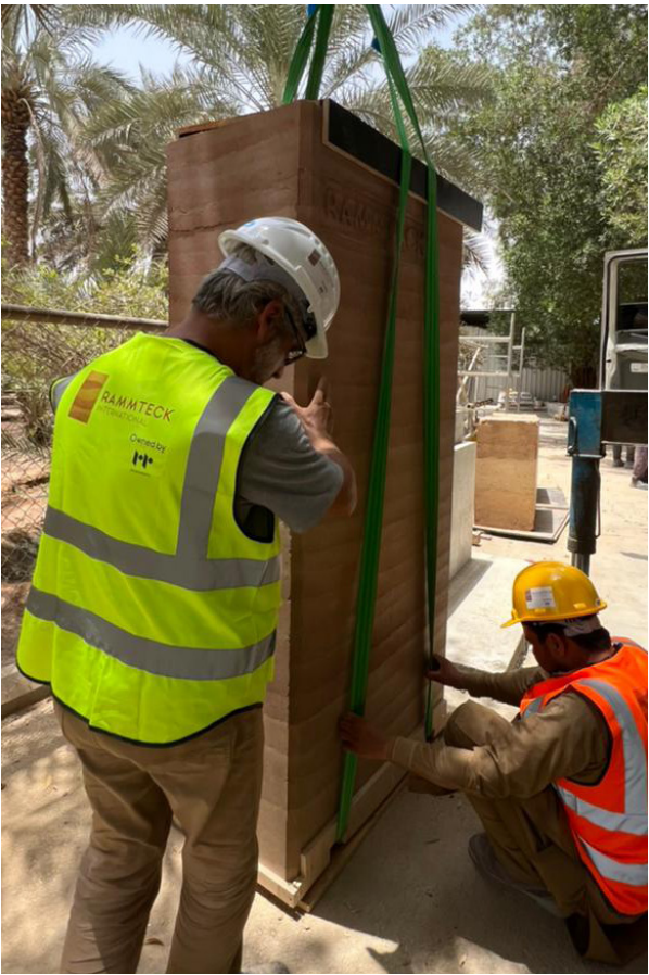
Fig 12.16 Rammed earth element: supported lifting straps
