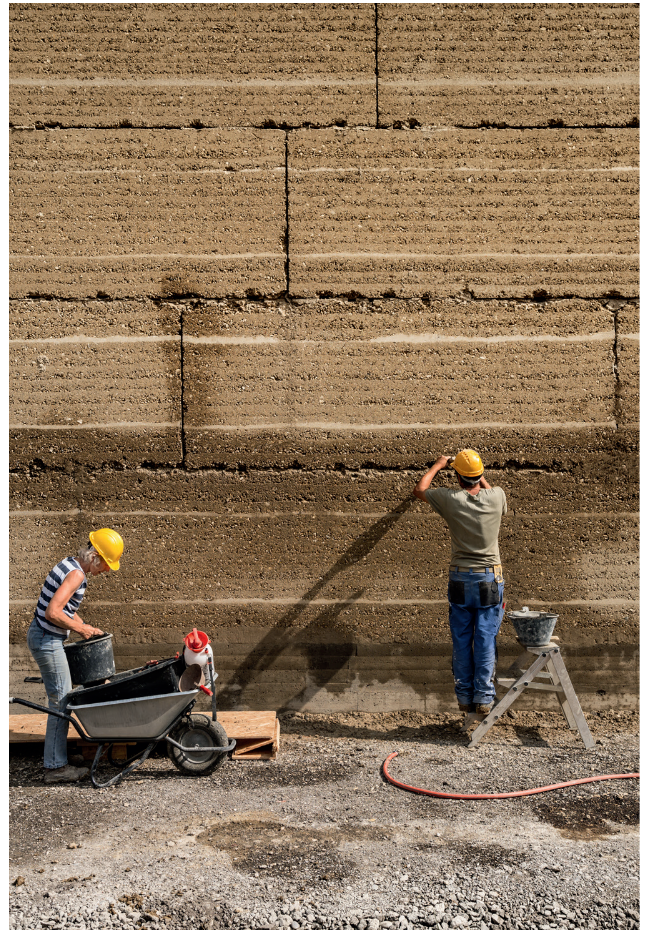
Fig 4.23 Workers finishing the gaps between the elements
