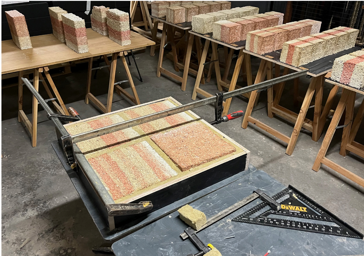
Fig 9.7 Constructing the frame, using two large bar clamps to clamp the panels, mineral wool and concreteplex together
