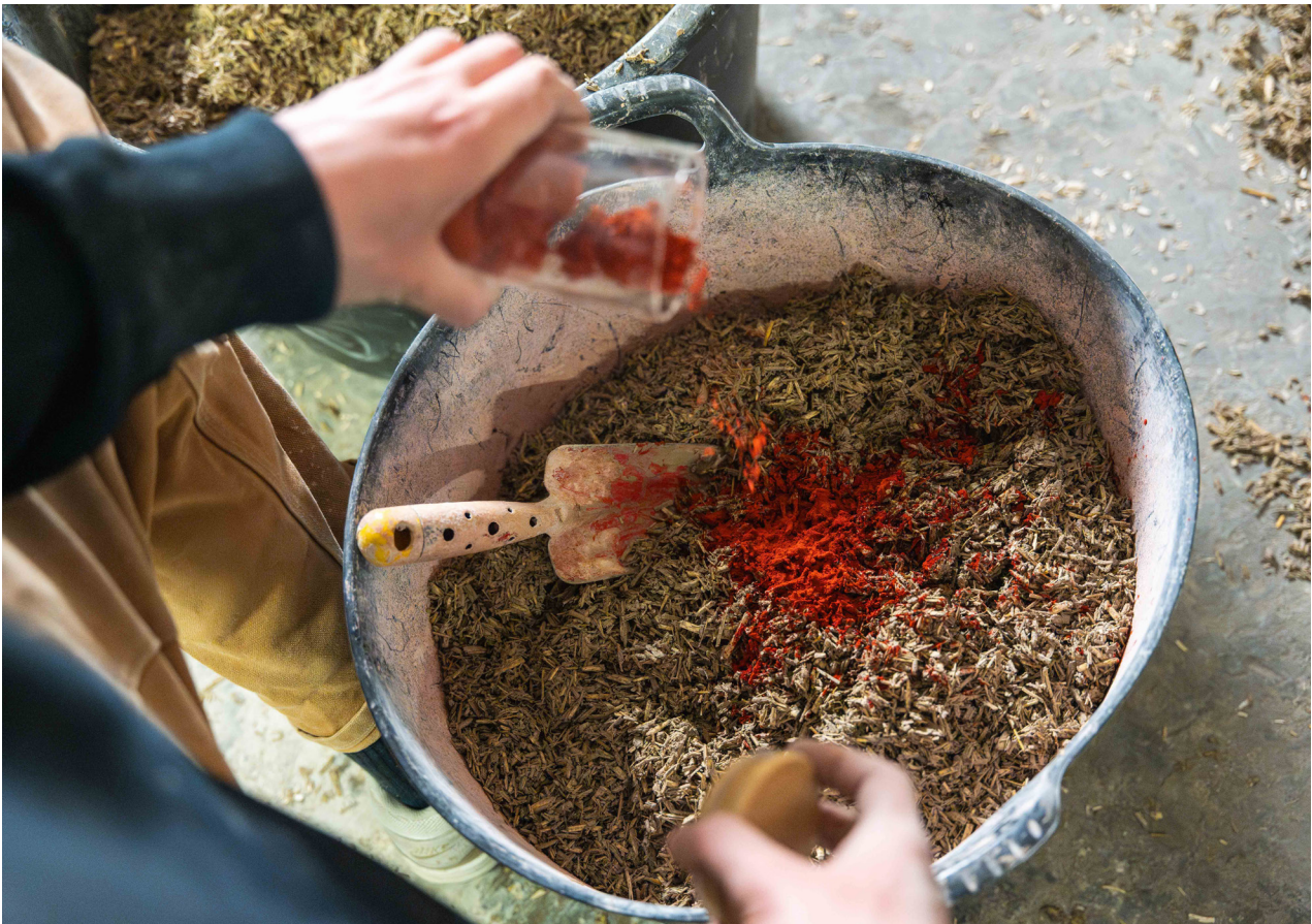
Fig 6.4 Adding pigment to the mix
