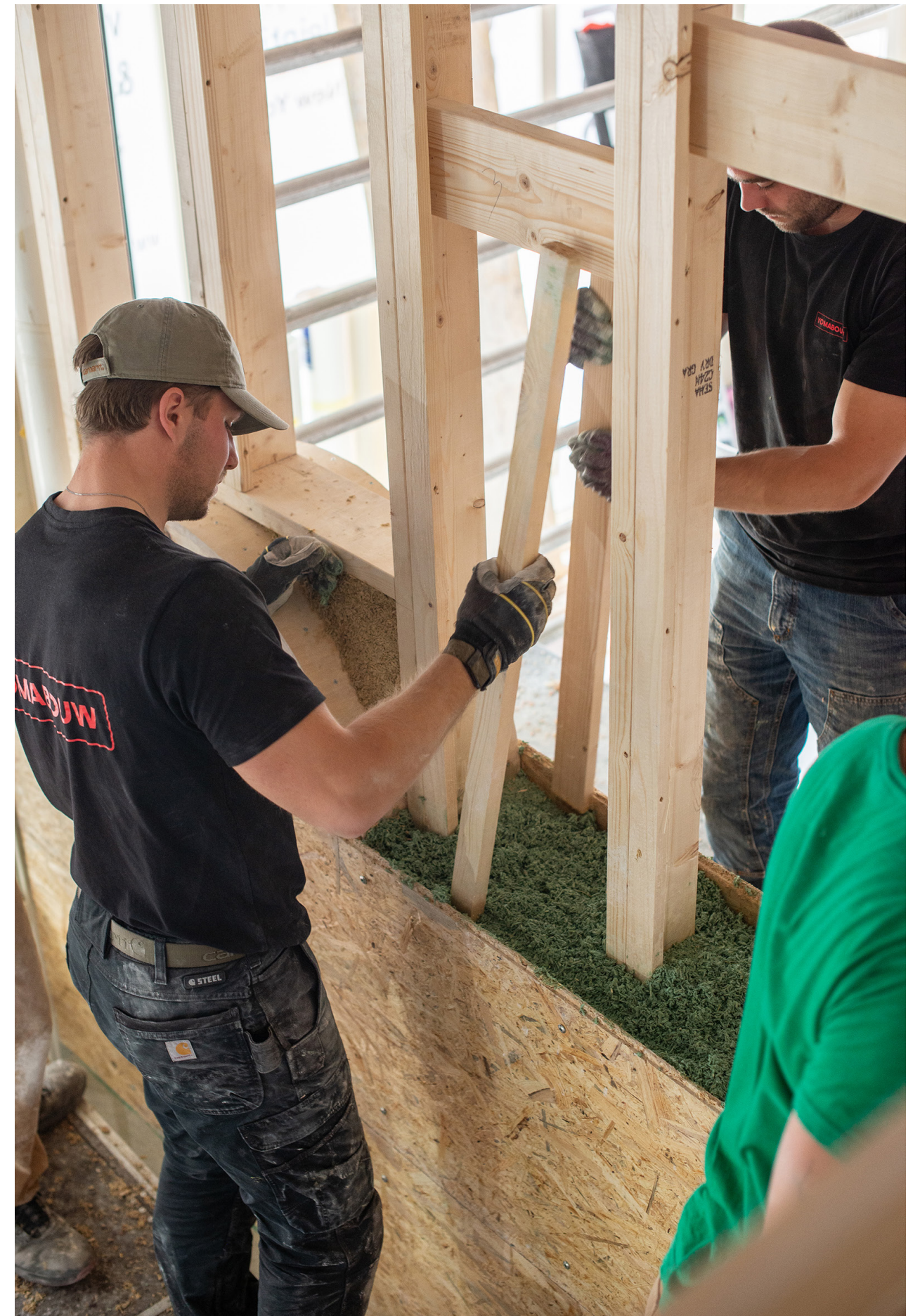
Fig 4.7 Manually tamping the sides with a wooden stick
