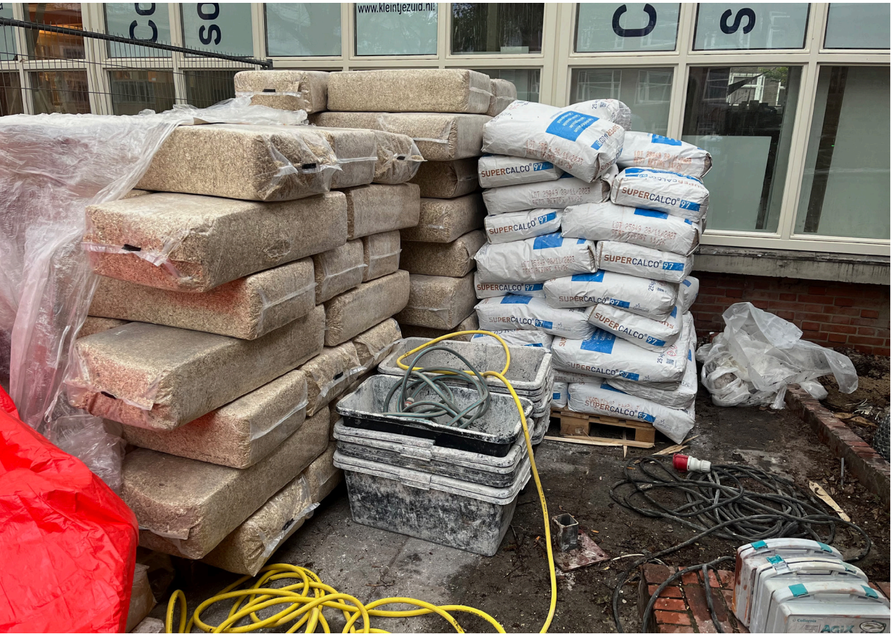
Fig 4.2 Hemp shivs, lime and mixing tubs on site
