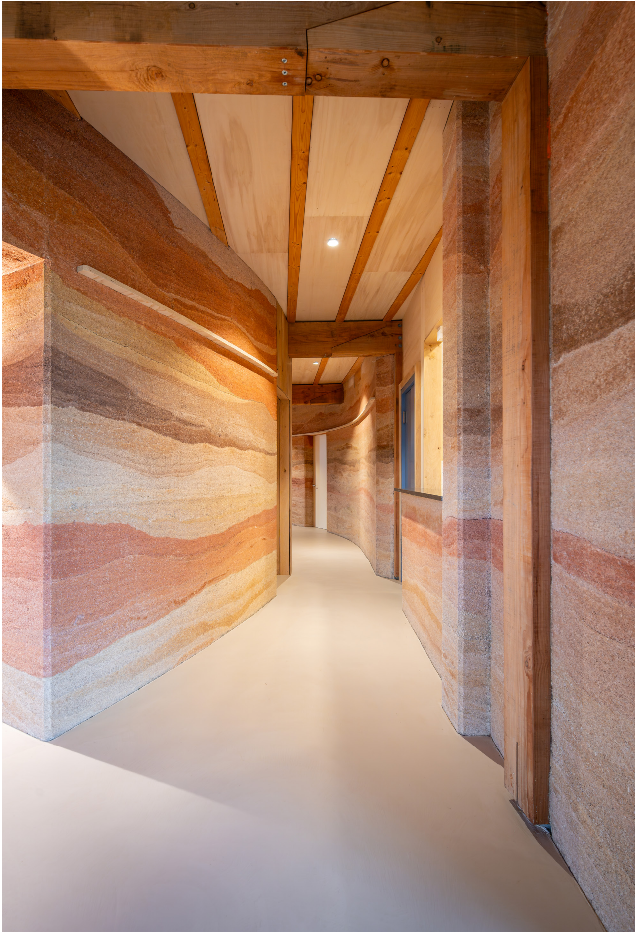
Fig 4.17 Cast-in situ hempcrete wall. Project by Giesen Architects and YOMABOUW
