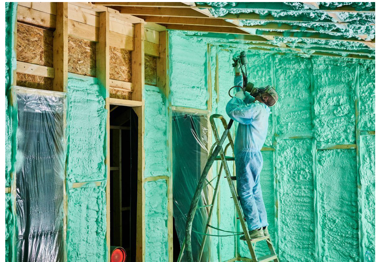
Fig 1.8 Worker insulation a home with toxic polyurethane foam, wearing a protective suit and mask against VOCs
