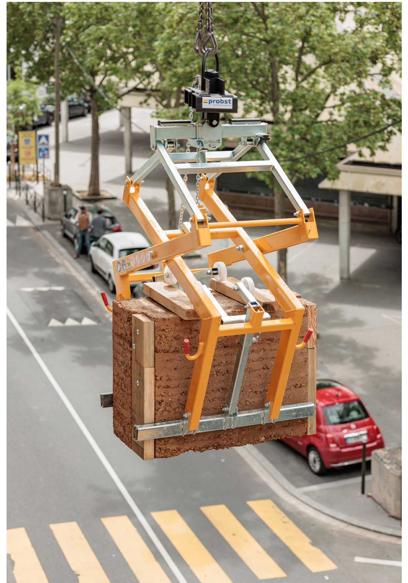
Fig 6.11 Craning Rammed Earth blocks into place on site
