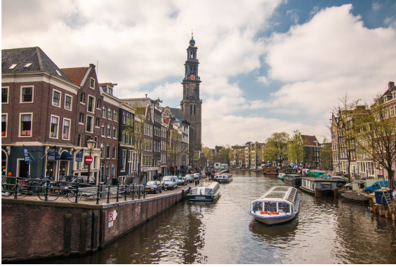
Fig. 1. Quay wall in Amsterdam.
