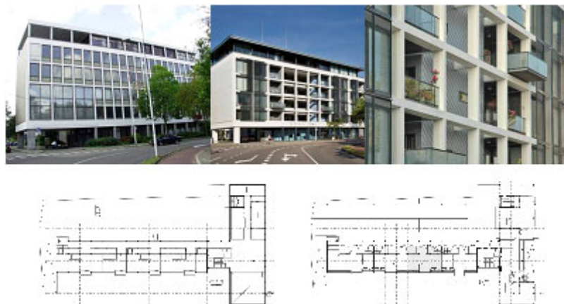
Figure 1 The Granida, one of the building transformations we studied ex-post. Left the office building before conversion, to the right the apartment building after conversion.
