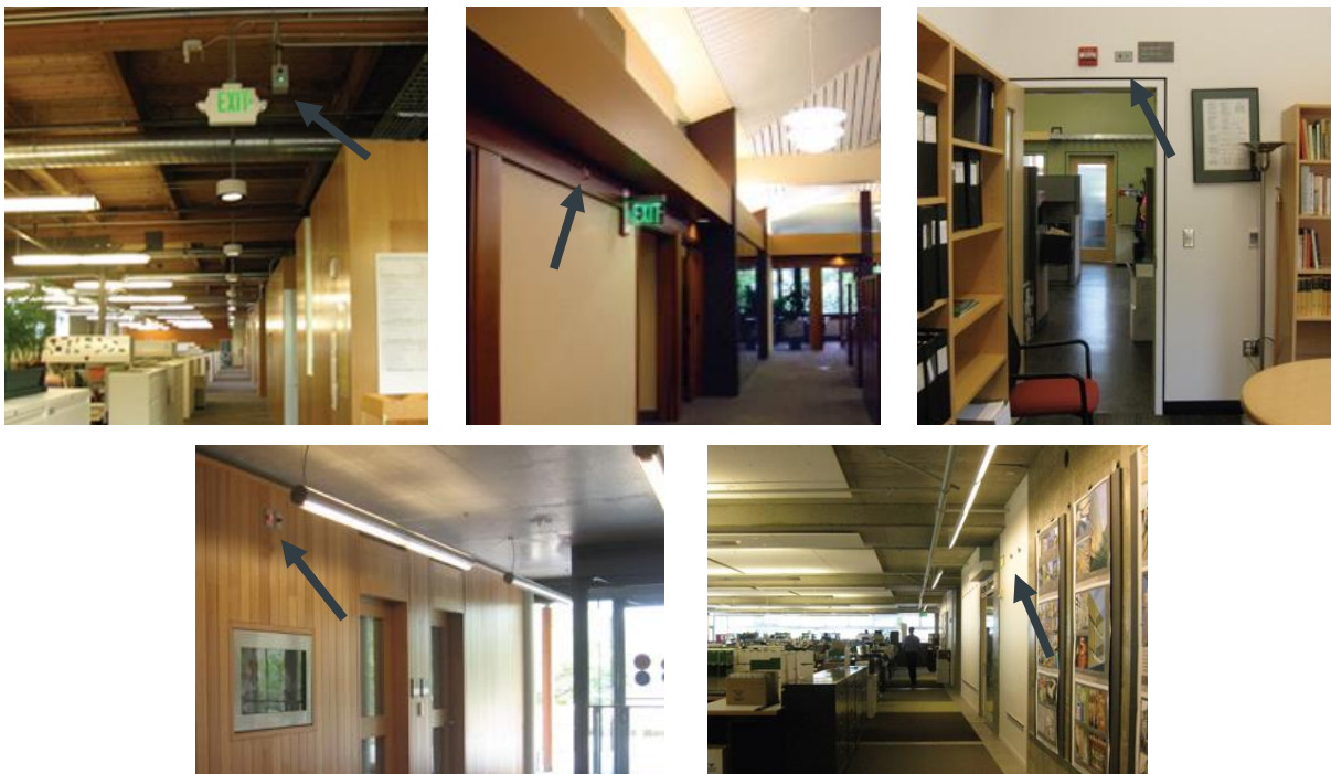
Figure 1: Encountered signalling devices by Ackerly and Brager which are not placed effectively and are easily overlooked when working. The shown signalling devices are placed far from the window and/or on the opposite side of the window (Ackerly & Brager, 2011)
