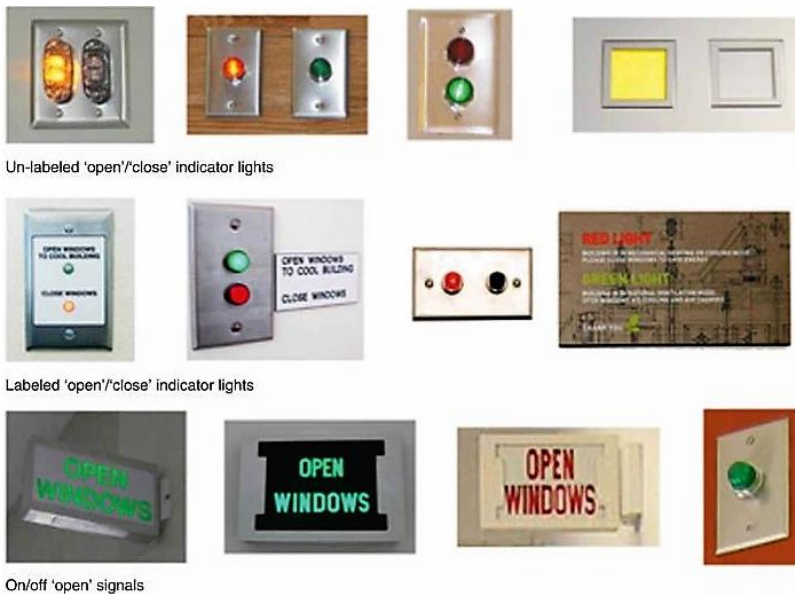
Figure 10: Different types of window signalling systems by Ackerly and Brager (2013)
