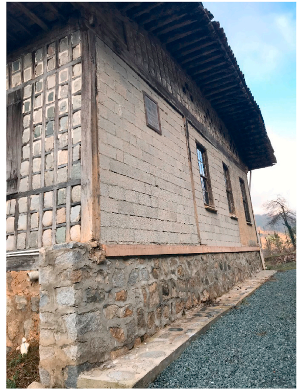
Fig. 9. The degradation of the rear façade of the Sevkety Atac House due to landslides in Çağlayan Village in Fındıklı of Rize. The photograph was taken by the first author, Gül Aktürk, on January 12, 2019.
