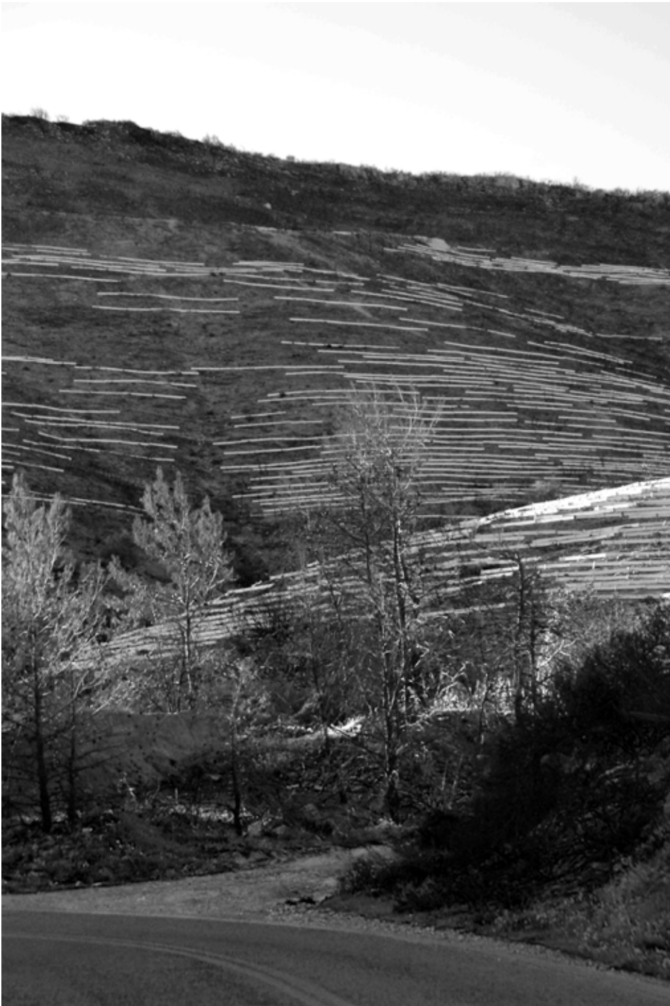
fig.46: Post-fire slope stabilisation with logs, Marathon, Greece
