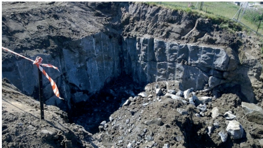
Controlled fracture by blasting
