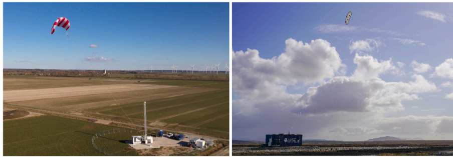
Fig. 3. The airborne wind energy systems in operation at the German site (left) and the Irish site (right). A drone captured the photo at the German site, while the photo at the Irish site was taken from the ground, differently affecting the perception of the kites' sizes (Courtesy of SkySails Group and Kitepower B.V.).
