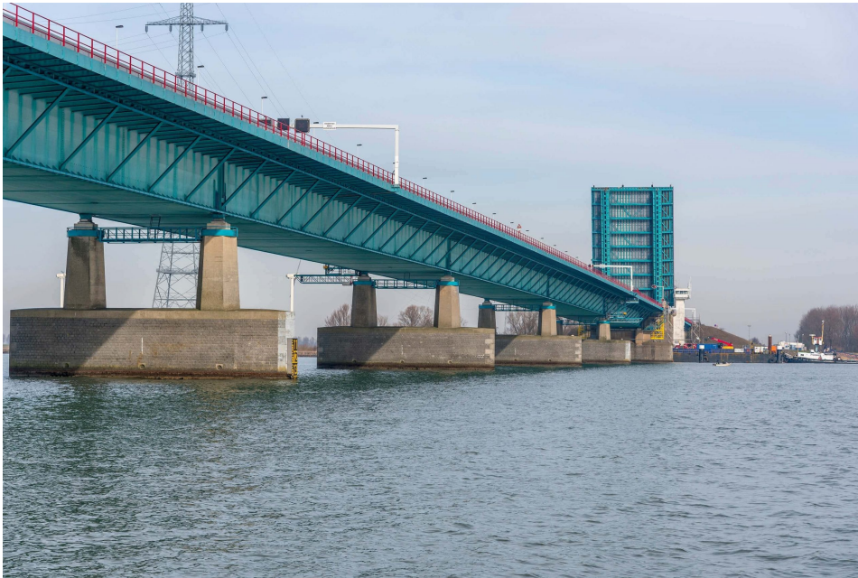
Figure 3.1: The Haringvlietbrug. Looking north at the drawn up moveable bridge. Source : Rijkswaterstaat
