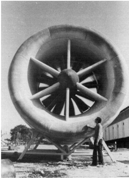
(a) The pilot plant DAWT of O. Igra ; the power generated is about 1 Kw at 5 m/s. [27]
