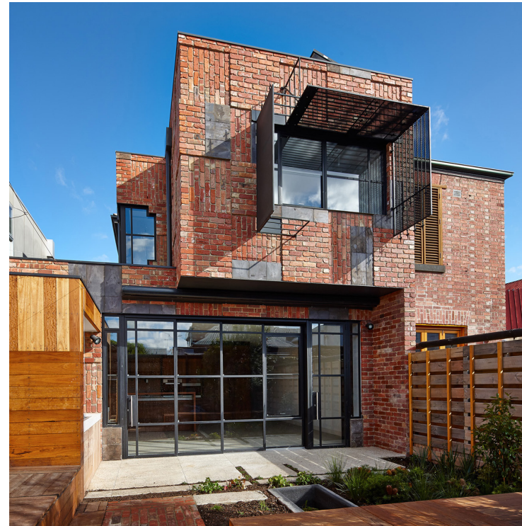
Cubo House - Phooey Architects
